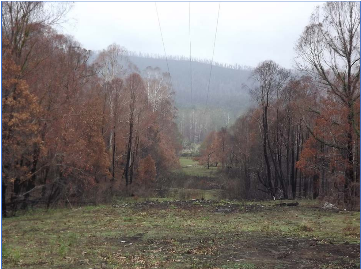
Figure 1: Powerline passing through burnt out forested landscape
