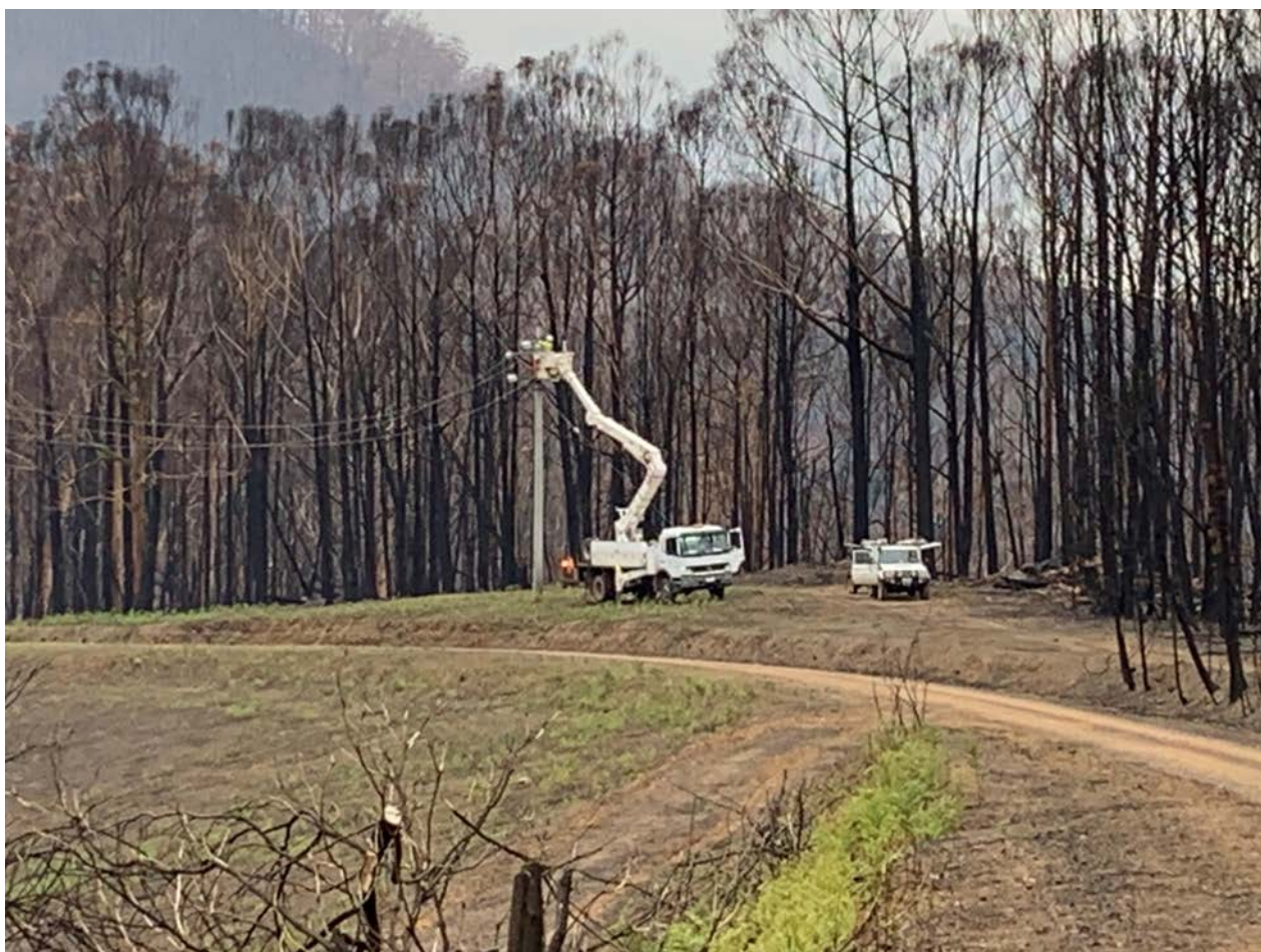
Figure 10: Powerline reconductoring work at edge of burnt forest
