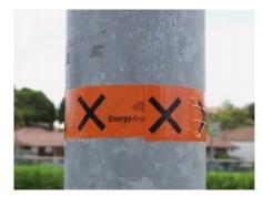
adhesive surface of the outer layer is evenly applied over the 1st layer, and not exposed to the air.
