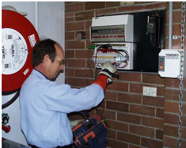
Figure 1 - Installation inspector tests a distribution sub board
