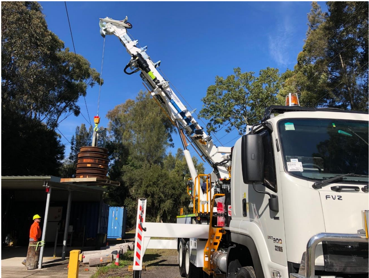
Figure 3 – Demonstration of Ozzy 6/10-16 Crane Borer in Hunter region.
