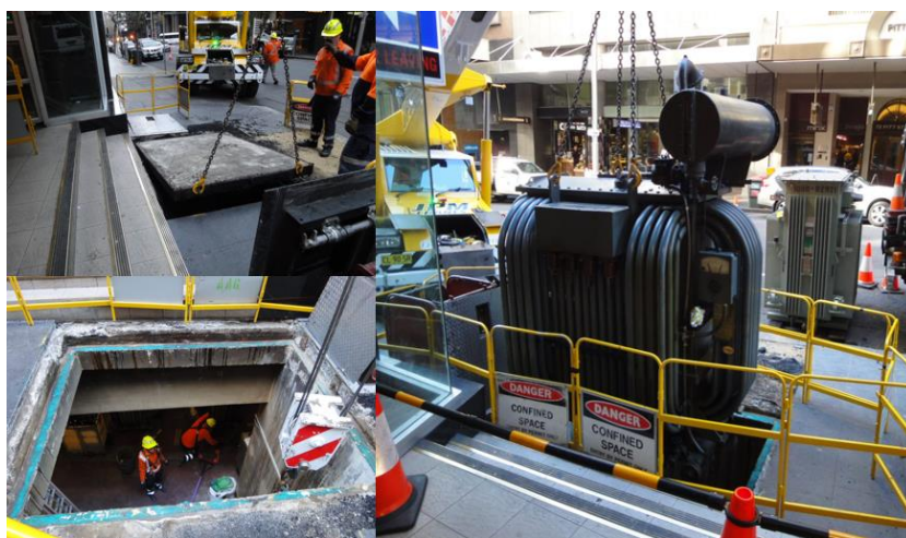
Figure 8: Images of the complex nature of CBD conservator-type transformer replacements
