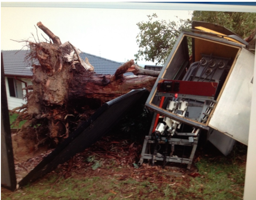
Image 2- Substation destroyed at Gateshead
