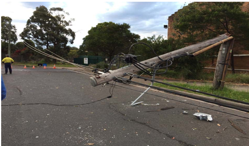
Image 5 (left image) Broken power pole at Rookwood
