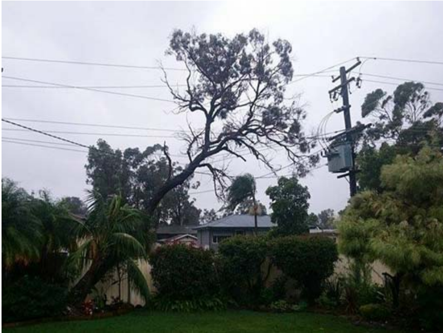
Image 1 - Tree on Wires at Berkeley Vale
