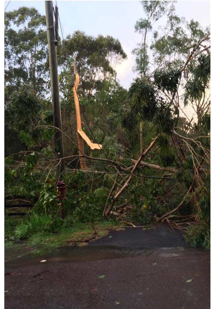
Image 4 - Fallen vegetation causing downed wires at Glen Road, Ourimbah
