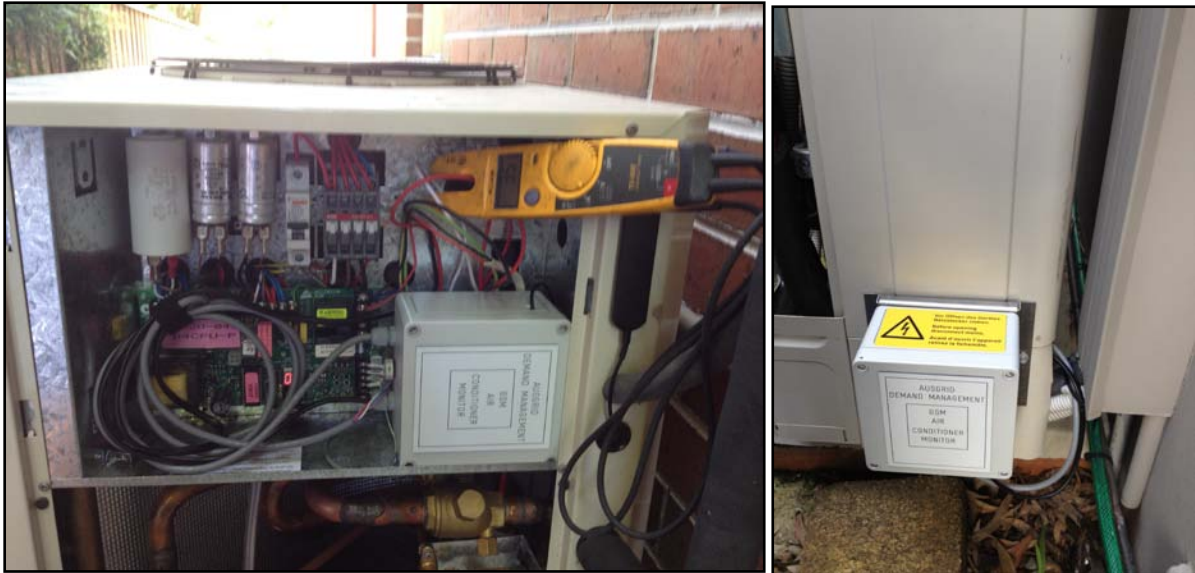
Picture: Two mobile phone DRED installations on air conditioners
