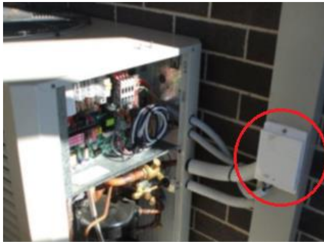
Figure –3G signal receiver (DRED) installed at test site
