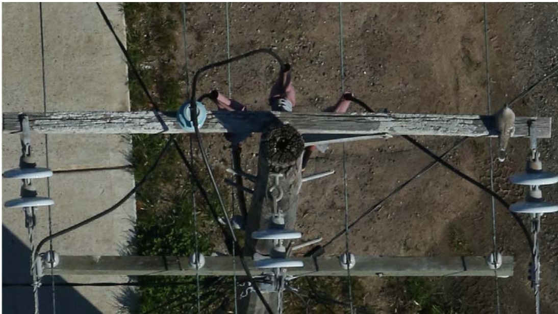
Figure 4. High definition image of a pole top, which can be reviewed for signs of asset defects.
