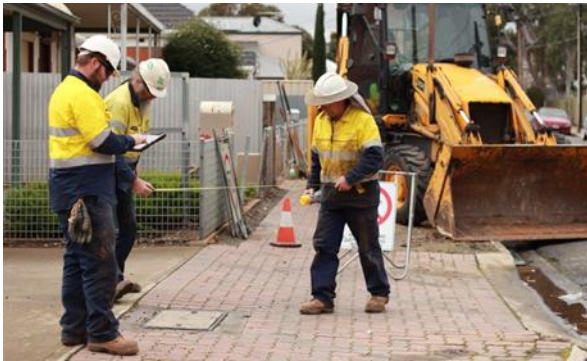
Response times – gas leaks
