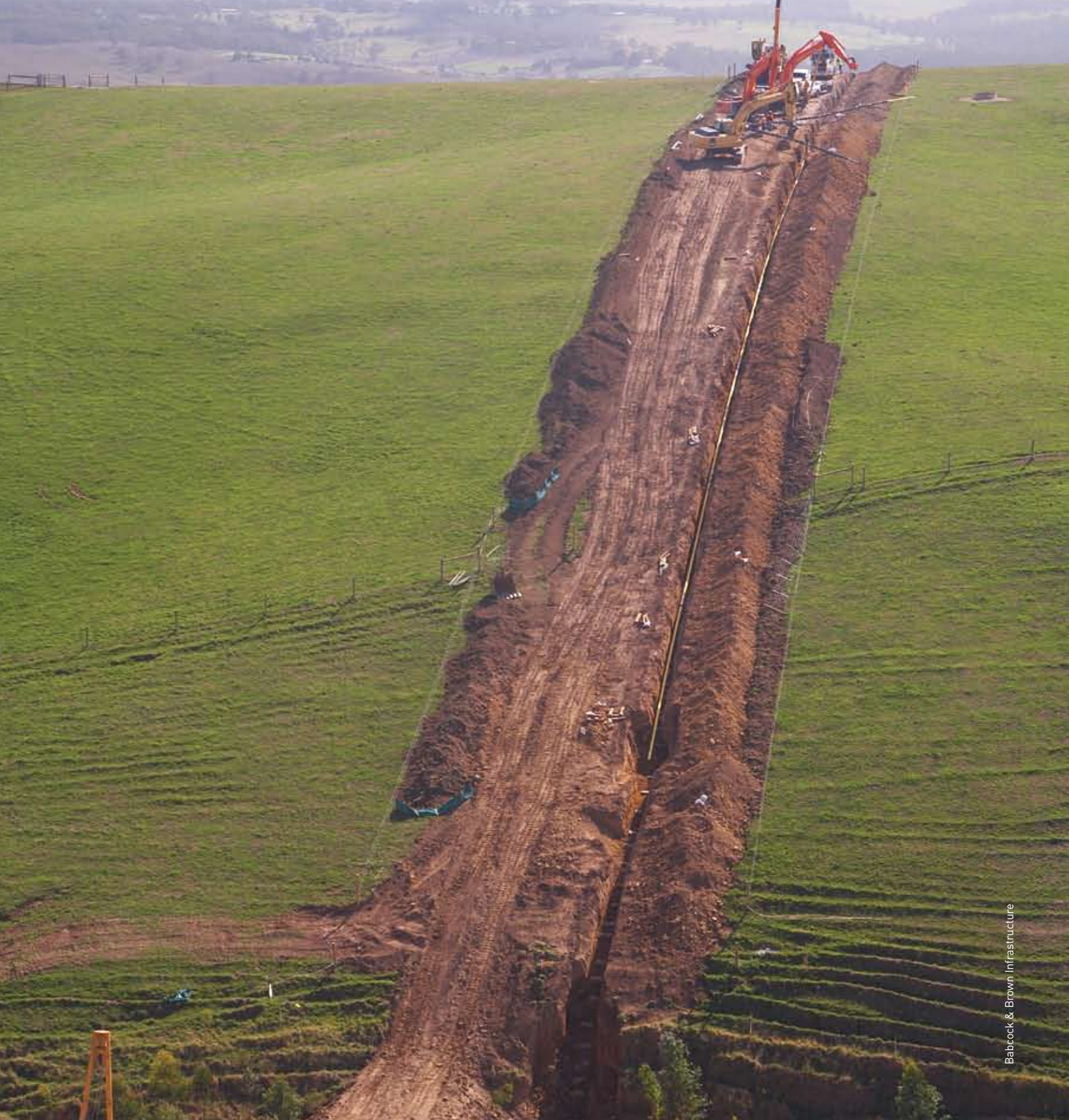
Construction of the South Gippsland Natural Gas Pipeline (Multinet)
