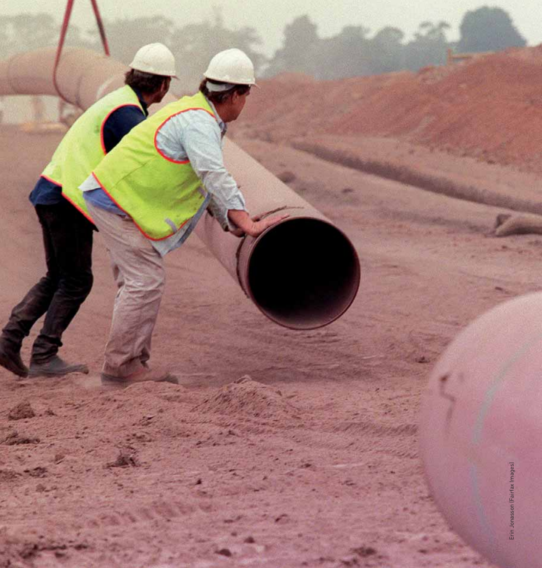
Laying of new gas pipeline
