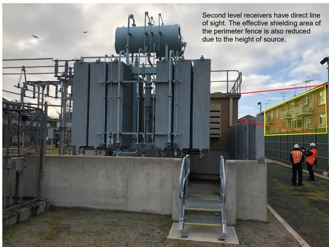
Figure 17 Example of reduced barrier performance
