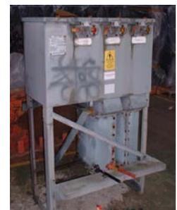
During RIIO ED 1 plan to replace RMU based on condition. We will be able to use our testing data and condition information to generate a prioritised plan. Units installed outdoors have suffered some deterioration due to corrosion dependant on location. In addition perishing gaskets, sight glasses, faulted barrier boards, damaged fuses, damaged contacts and internal corrosion have informed our investment assumptions for such assets.
