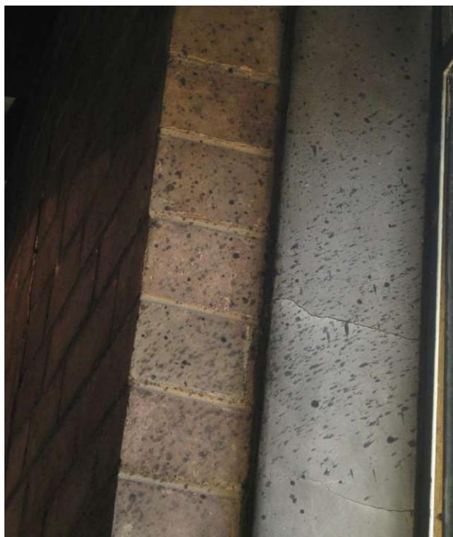
Figure 2: Evidence of hot oil spray from a failed switchgear
