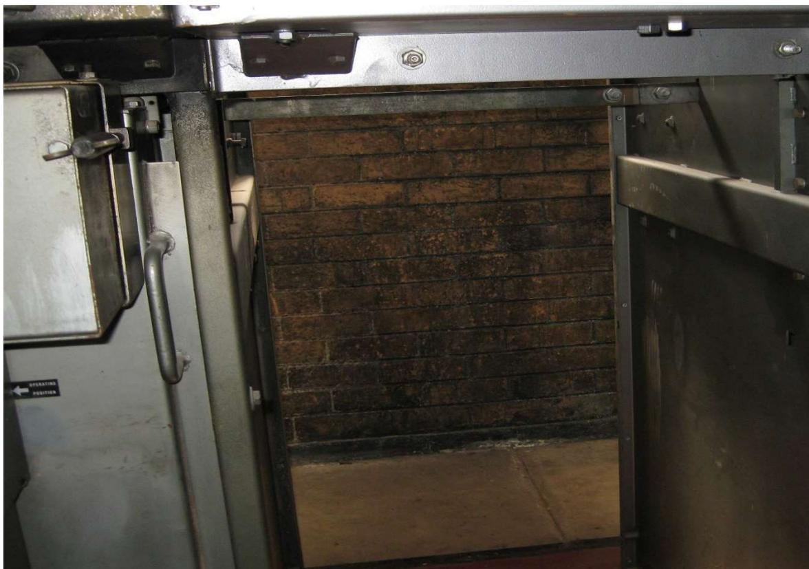
Figure 1: Evidence of explosive switchgear failure at WD
