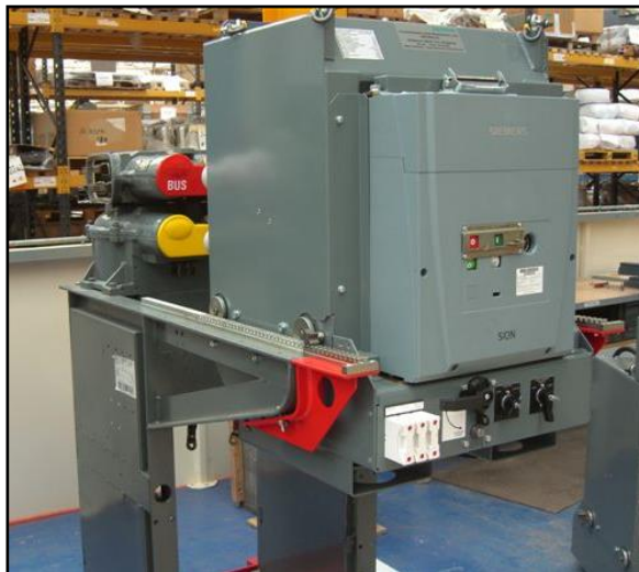
Figure 21 – Siemens Sion-C Retrofit CB
