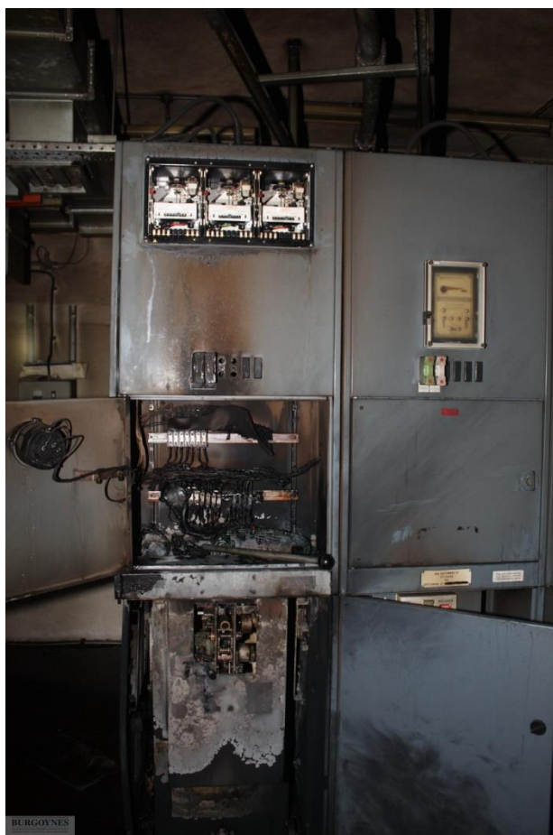
Figure 18 – GEC VMX: Failed 11kV panel
