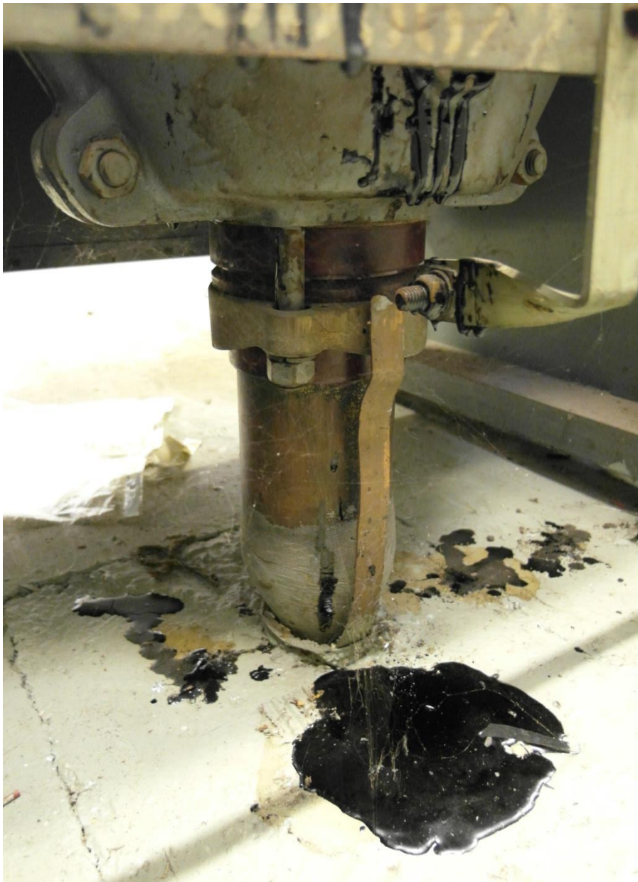
Figure 7 – Typical compound leak from a cable box
