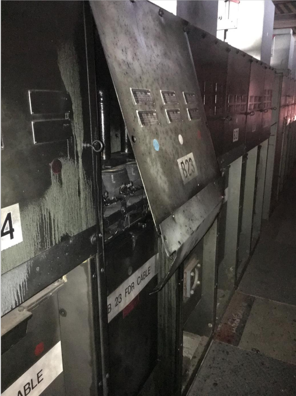
Figure 5 Damage to rear of air-insulated busbar chamber and switch room due to uncontained arc fault
