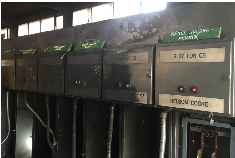
Figure 3 Damage to B switchboard and switch room following circuit breaker failure
