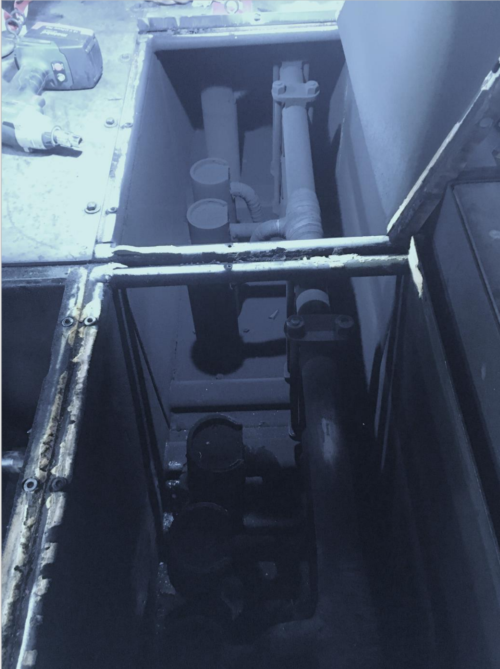
Figure 4 Damage to B no.4 busbar following circuit breaker failure
