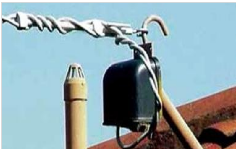
Figure 4.4 Sample image: twisted PVC service line
