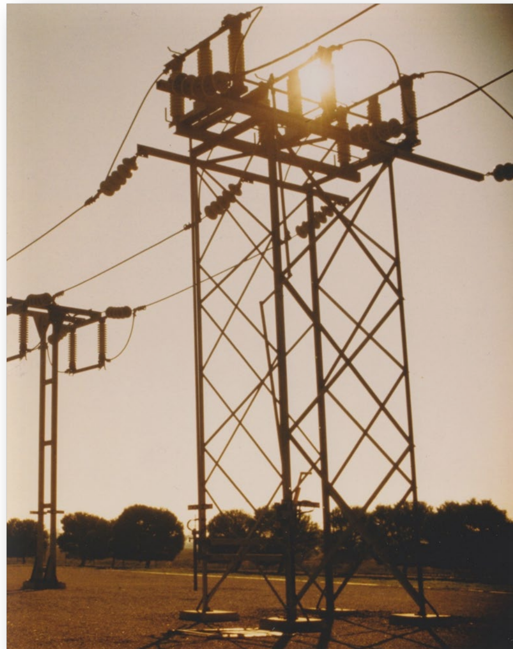
Photo: 66kV switch, Powercor, 1997
