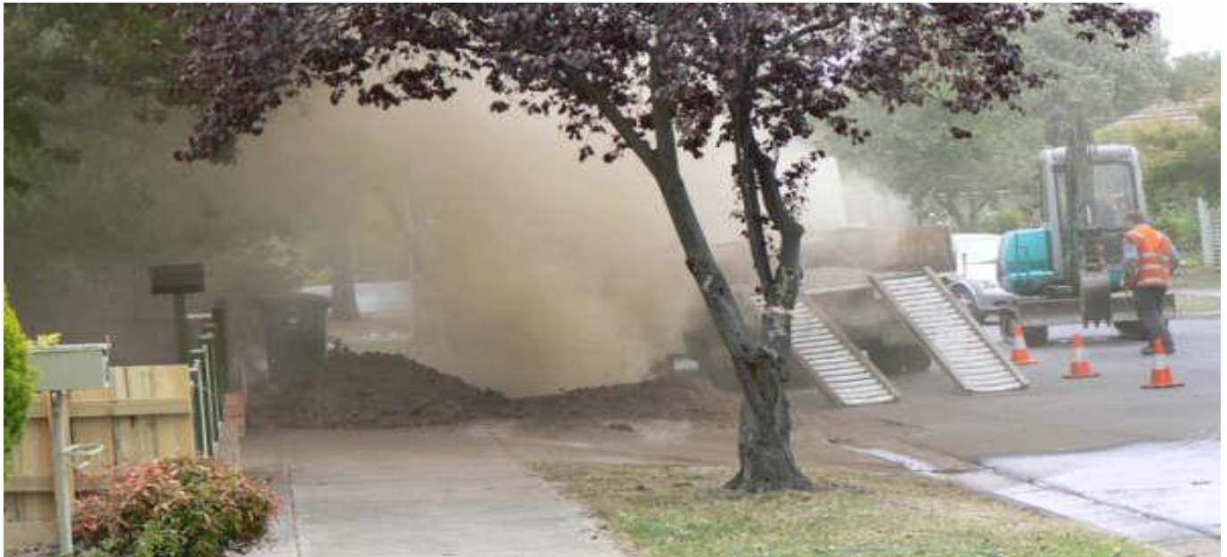
Figure 13-1: A large diameter Medium Pressure escape
