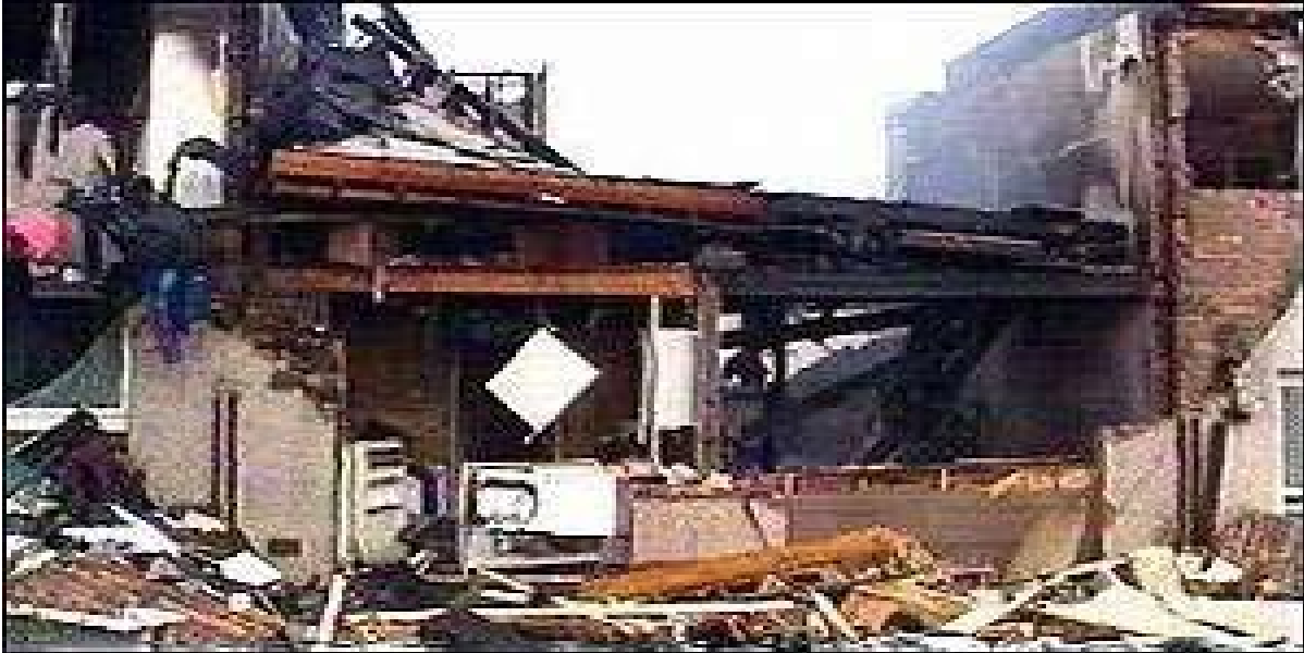
Figure 13-2: Damage to a House (Dundee UK 1990)
