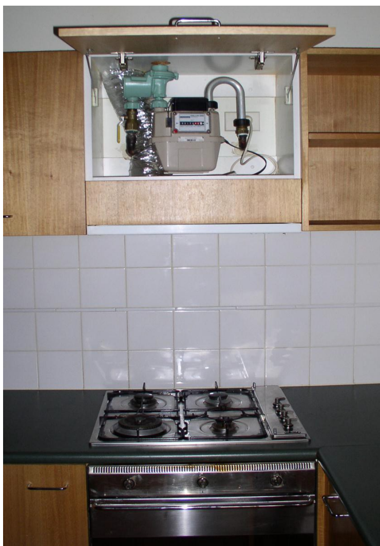
Figure 13-10: A Hexagram meter inside an overhead cupboard above hotplates and adjacent to a power point.
