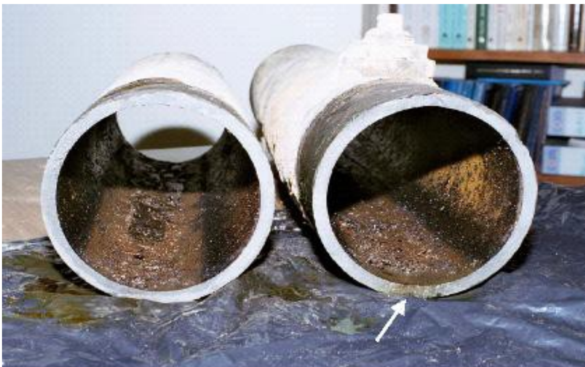
Figure 13-3: Fracture Failure Mode
