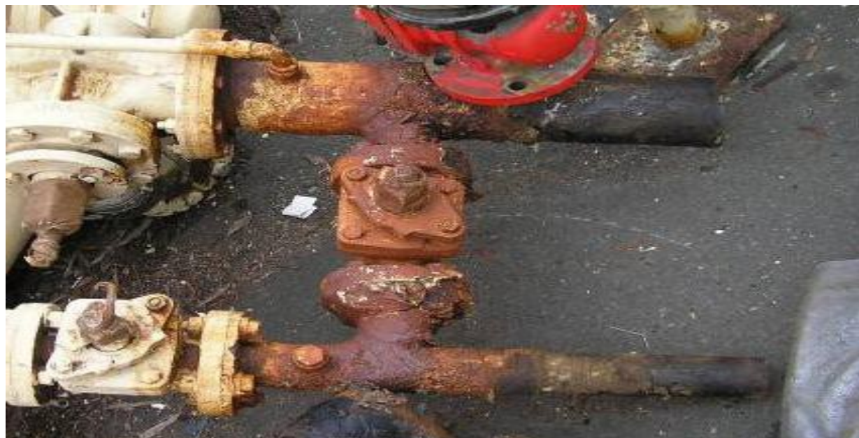
Figure 13-9: Typical Corrosion on Trombone Style Regulator
