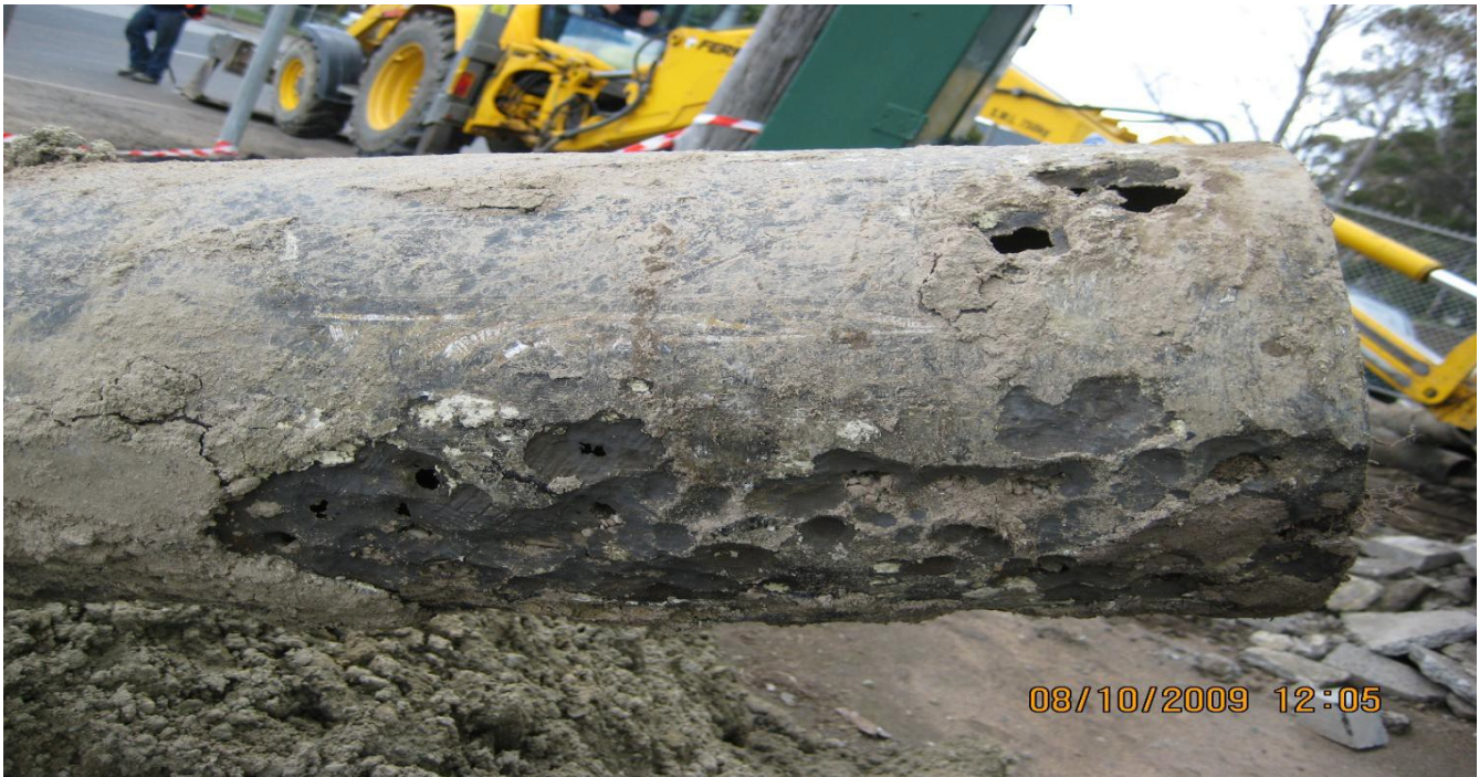
Figure 13-8: Severe Corrosion on 225mm uncoated steel pipe
