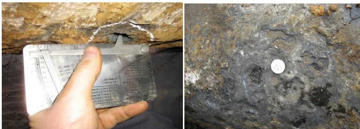
Figure 13-5: Wall Thickness Loss
