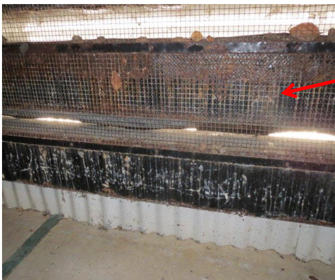
Internal View of corrosion in building
