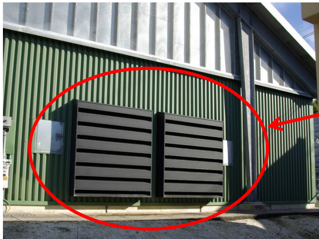
External View of building sound dampers
