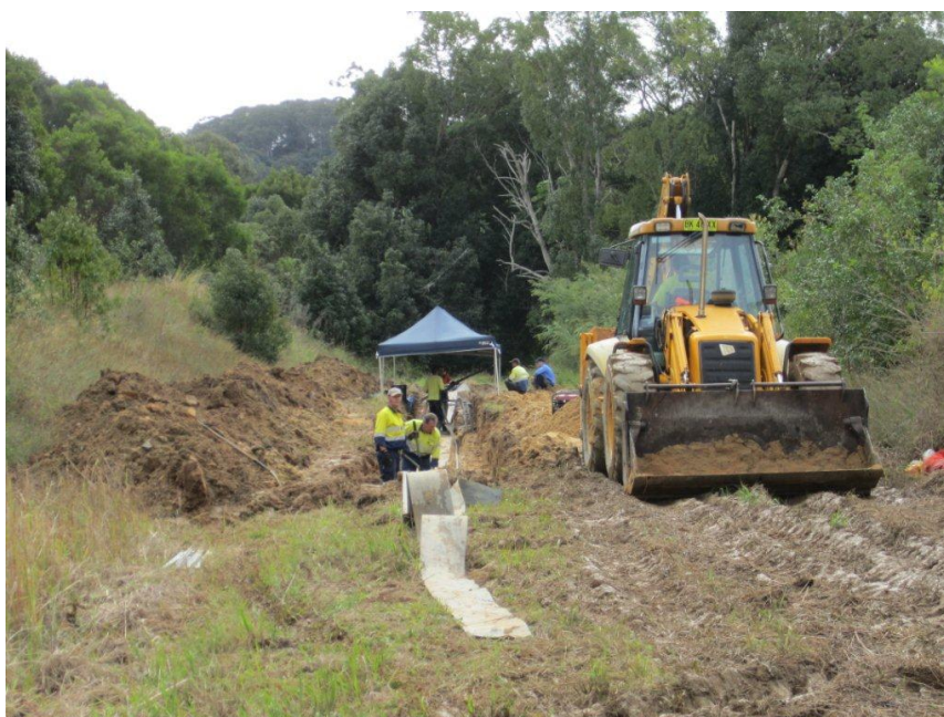
Figure 13: Photograph taken during an underground cable repair
