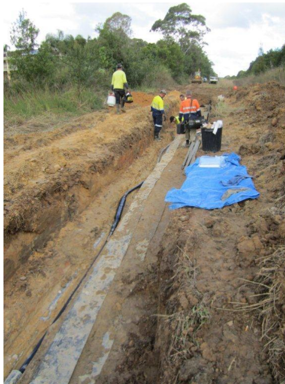
Figure 14: Covering the cables with barrier tape after a cable repair
