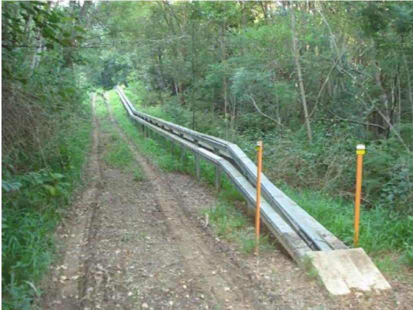
Figure 1 - Typical Directlink GST and Transition
