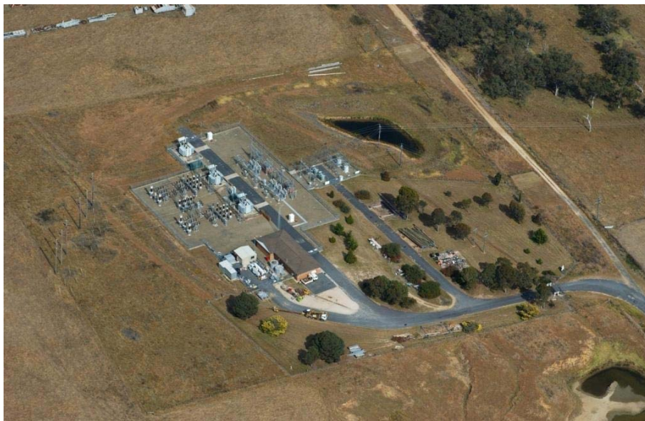
TENTERFIELD 132/22/11KV SUBSTATION.
