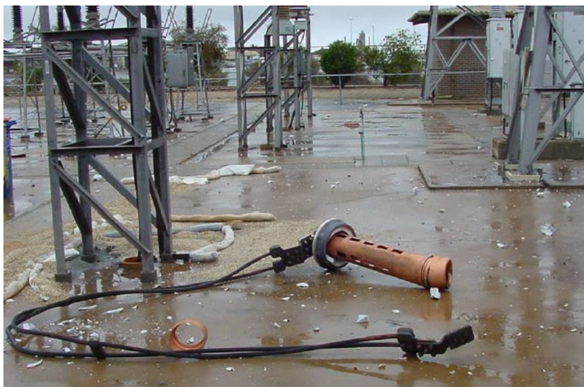
Figure 9: Porcelain Circuit Breaker Explosive Failure
