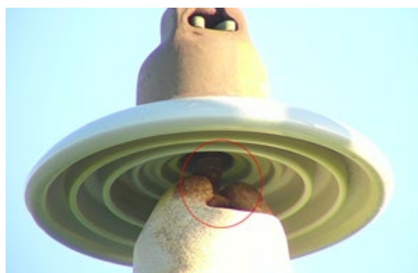
Figure 3: Line Insulator Pin Metal Loss Due To Corrosion
