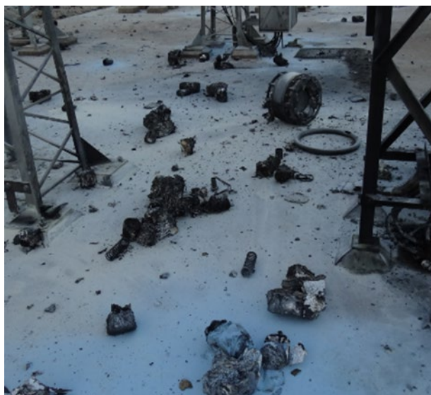
Figure 7: Instrument Transformer Explosive Failure
