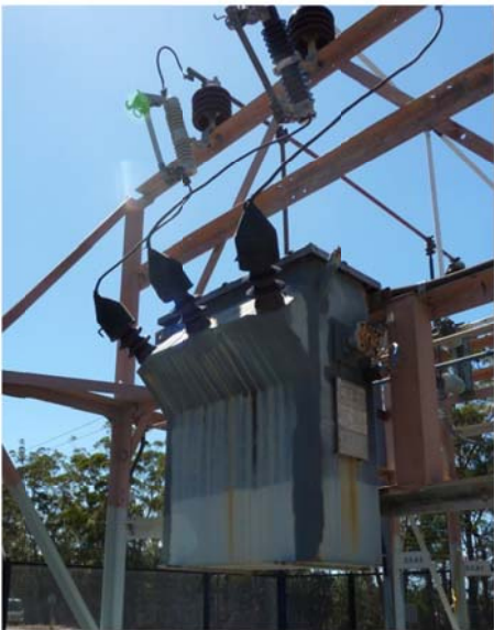
11kV auxiliary transformer
