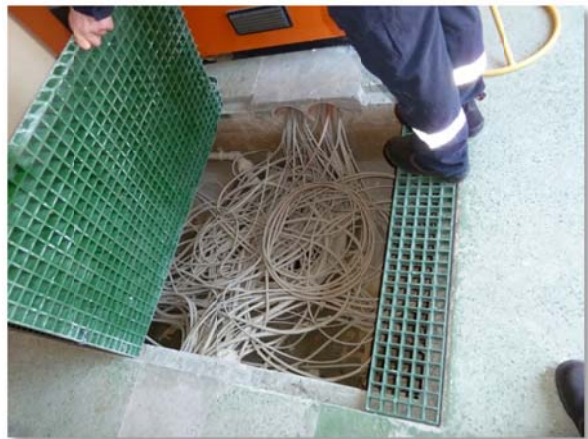
Control building with damaged roof and cable pit subject to flooding
