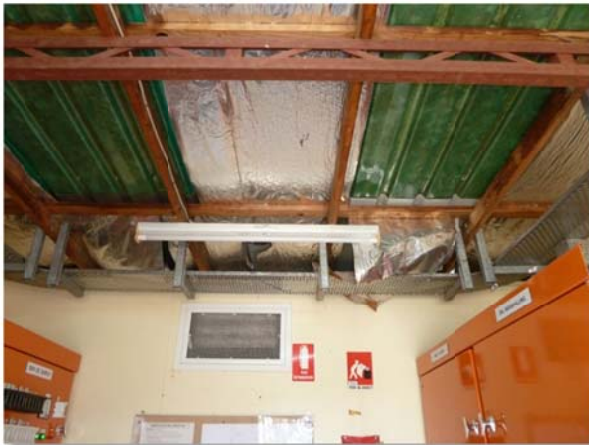
Control building with damaged roof and cable pit subject to flooding
