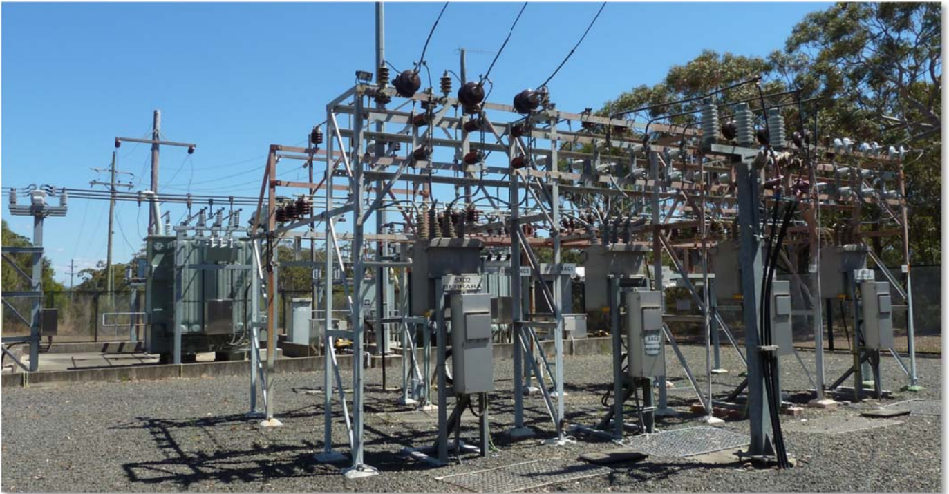
Sussex Inlet ZS showing the 11kv busbar structure and the four feeder reclosers
