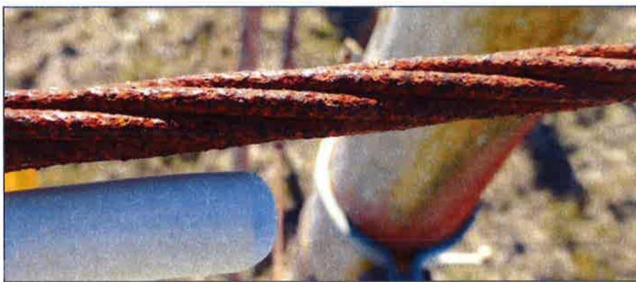
FIGURE 3 : FEEDER 941 – EARTHWIRE IN CATEGORY 4 CONDITION
