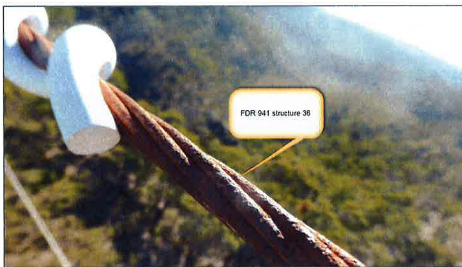
FIGURE 3 : FEEDER 941 – EARTHWIRE IN CATEGORY 4 CONDITION
