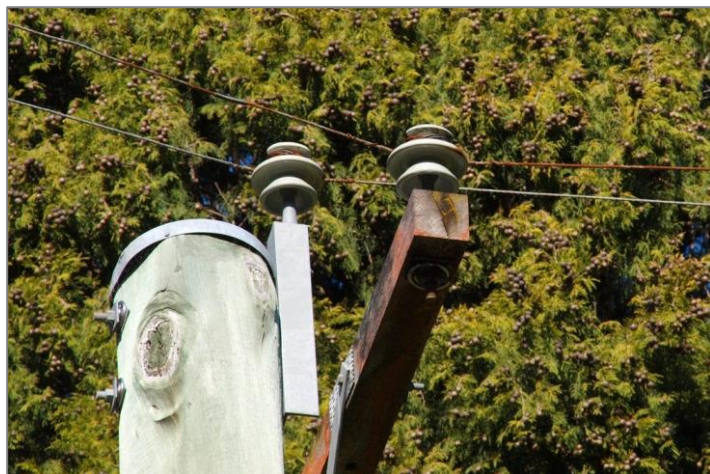
FIGURE 1 - CORRODED 7/0.064 SC/GZ CONDUCTOR IN SERVICE AT LEURA
