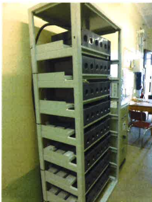
120 VDC battery bank
