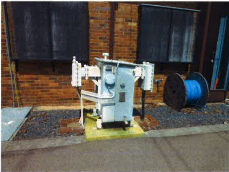
Auxiliary transformer – slight oil leak from tap changer
