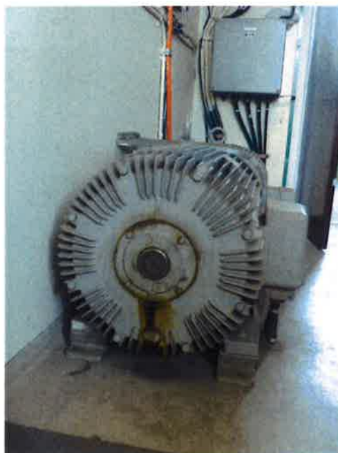
Motor generator set oil leak from motor side
