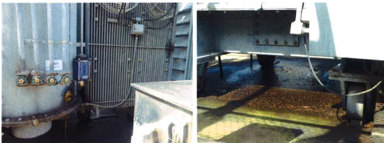
Tyree 33kV/11kV 25 MVA TX no. 1 oil leak from radiator and tap changer
