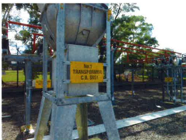
TX no. 1 33kV CB – Hawker Siddeley Horizon (installed 2011)
