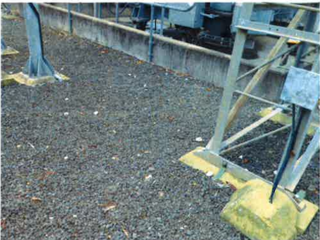
Stones (white) and other foreign material was found scattered in the switchyard near power transformers and 33kV outdoor circuit breakers
