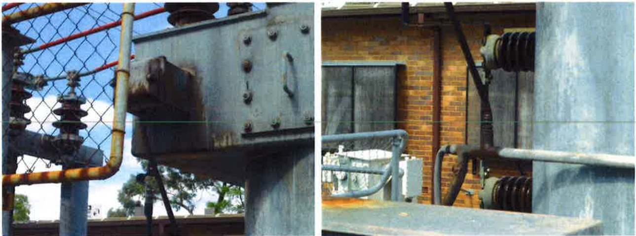
Tyree 33kV/11kV 25 MVA TX no. 2 – oil leak from RTD box
