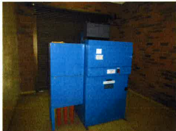
11kV Bulk oil Reyrolle LMTs Power TX secondary side circuit breakers
