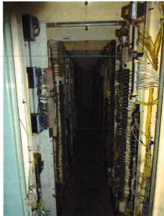
Tunnel boards (old design - all exposed terminations)
