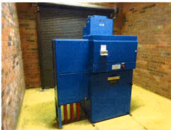
11kV Bulk oil Reyrolle LMTs Power TX secondary side circuit breakers
