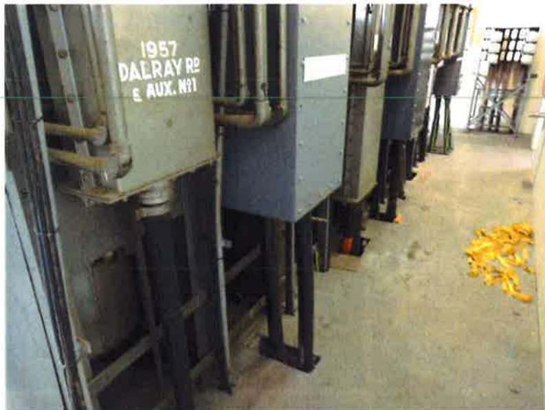
11kV Westinghouse B18 breakers (rear view)
