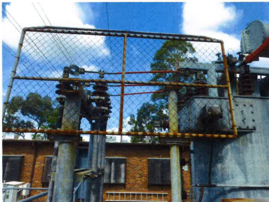
Tyree 33kV/11kV 25 MVA TX no. 2 – rust and surface corrosion on structures
