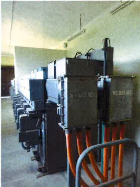
11kV Westinghouse B18 breakers
