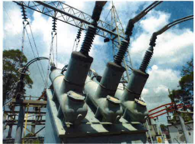
Feeder 473 33kV CB – Alstom OX36 (installed 2004)
