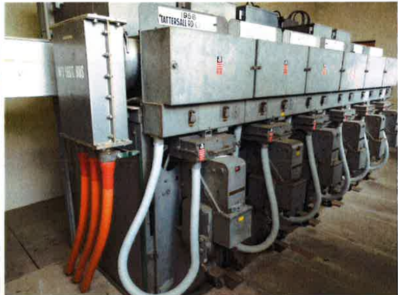
11kV Westinghouse B18 breakers arc chute and closing coil contactor covers contain asbestos
