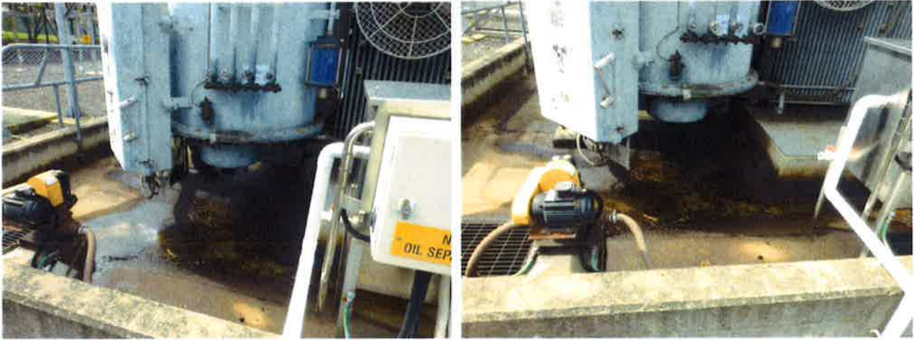
Tyree 33kV/11kV 25 MVA TX no. 2 – oil leak from gaskets
