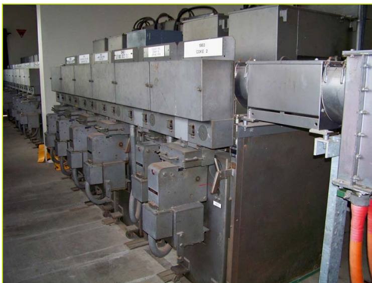
11kV Westinghouse B18 switchgear
