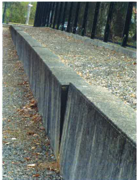
Retaining wall is slanted
