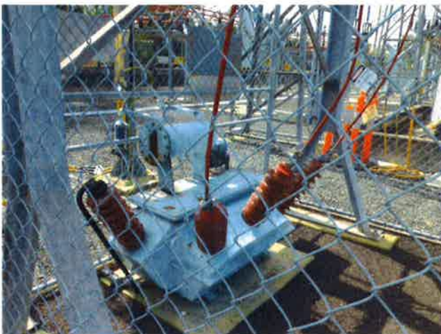
33kV 3-phase Voltage Transformer – Hanson
