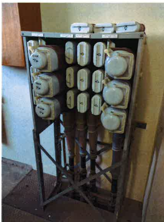
Holec MD4 auxiliary switchboard
