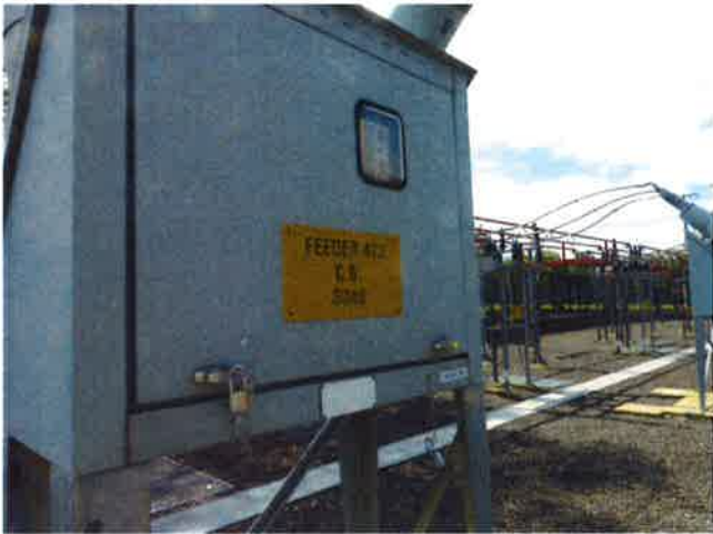
Feeder 473 33kV CB – Alstom OX36 (installed 2004)
