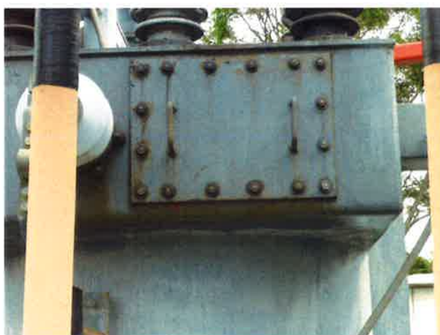
TX no. 1 oil leak from top bushing gaskets
