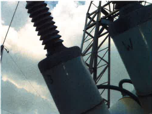
Bushing weather shield and denting on bushing turrets on Alstom 33kV OX36 CBs
