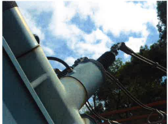
Bushing weather shield and denting on bushing turrets on Alstom 33kV OX36 CBs
