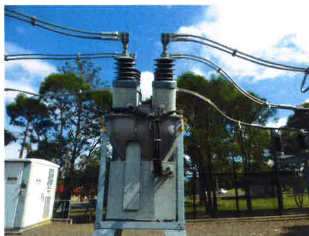
TX no. 1 33kV CB – Hawker Siddeley Horizon (installed 2011)
