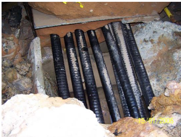
Bottom Right – Feeder 22W & 233 (ground subsidence and debris impacting cables after water mains failure in 2007) - 2007
