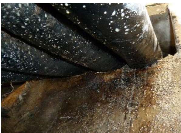
Bottom left – Feeder 9J8 (leaking oil at bridge crossing in Rosehill) - 2013
