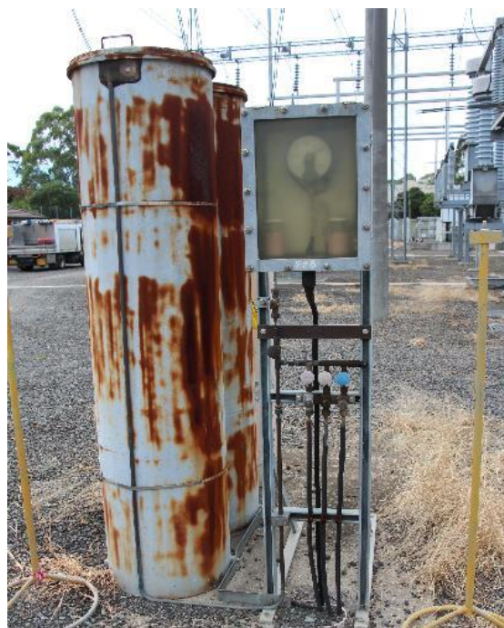
Top Right – Feeder 228 at Guildford TS (severely corroded oil reservoir tanks prior to TM302) - 2017
