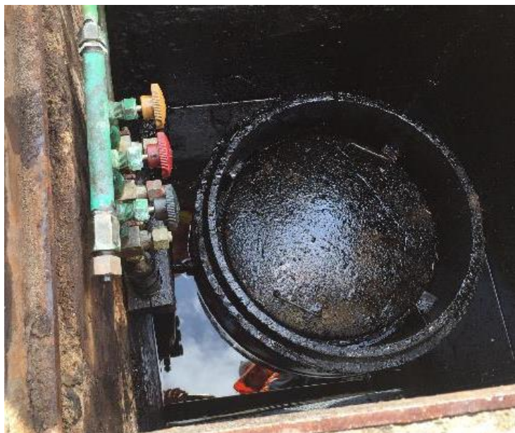
Top Left – Feeder 228 joint bay 4-5 (cable oil in base of joint pit) - 2017
