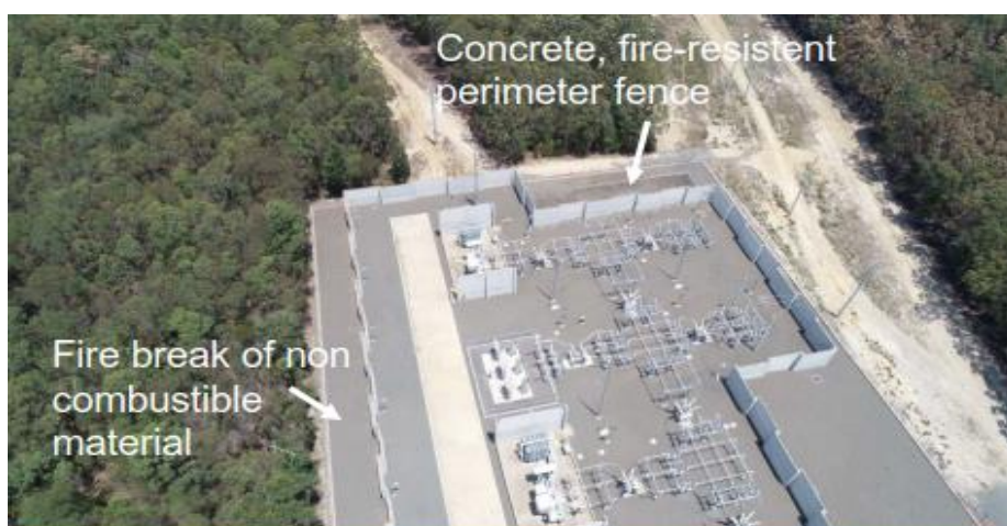
Figure 4 - Bushfire mitigation features of Tomerong sub-transmission substation
