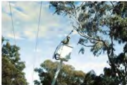
Tree trimming to maintain safety clearances, prevent outages from branches and trees falling on power lines, and to reduce the risk of bushfires
