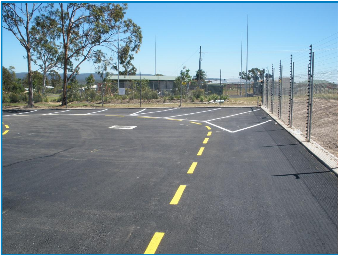
Image 17: New improved hardstand, driveways, parking areas and security fencing.
