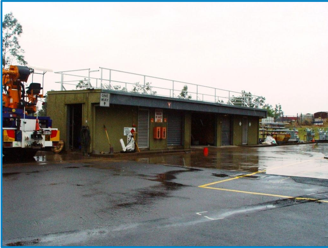
Image 16: Gatton hardstand and driveway area prior to works.
