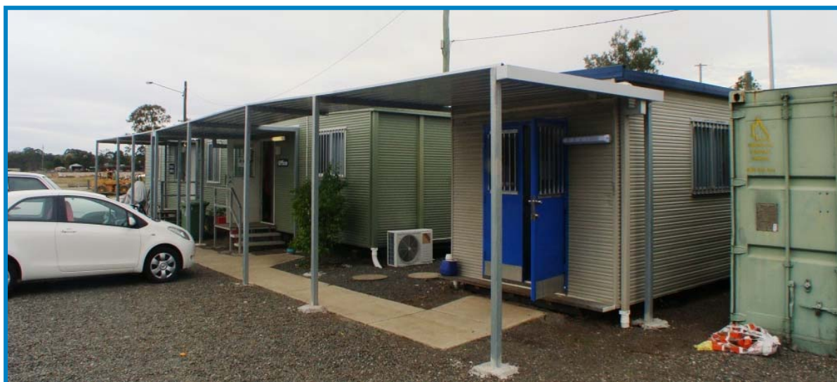
Image 2: Original office set-up in demountable buildings at the Landsborough Depot prior to CPS works.
