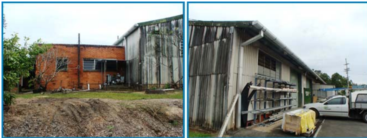
Image 6: The aged, dilapidated former Energex depot facility at National Park Road, Nambour.
