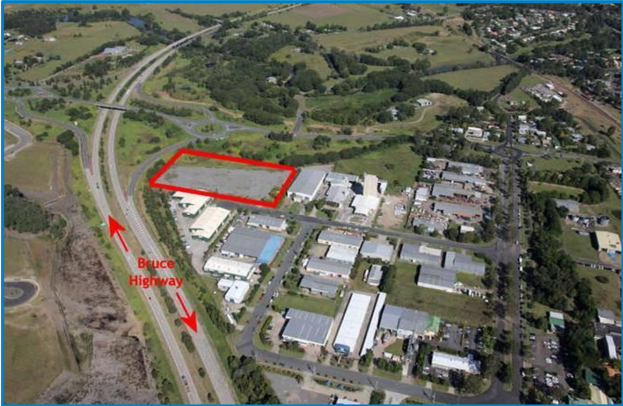
Image 12: Location of Yandina Depot is ideal due to access to Bruce Highway, servicing the North Coast region.
