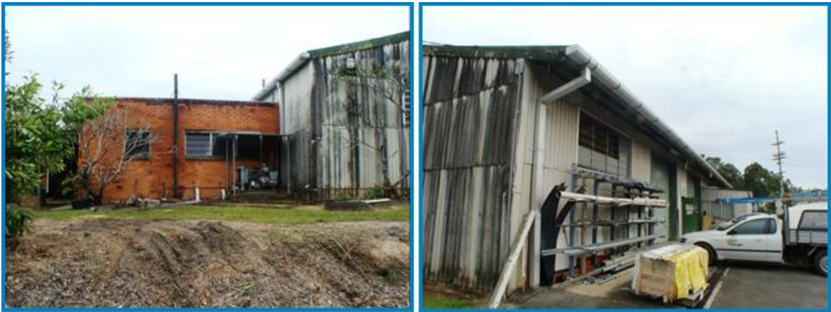
Image 13: The aged, dilapidated former Energex depot facility at National Park Road, Nambour.
