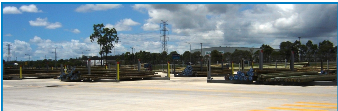
Image 1: Pole & cable yard at Southern Distribution Depot, Larapinta, a CPS project, completed July 2011.
