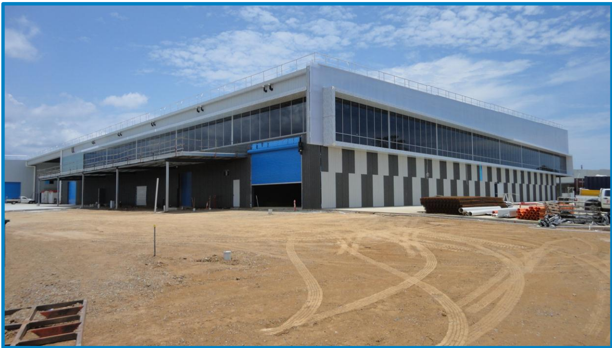
Image 3: The Geebung Redevelopment Project underway.
