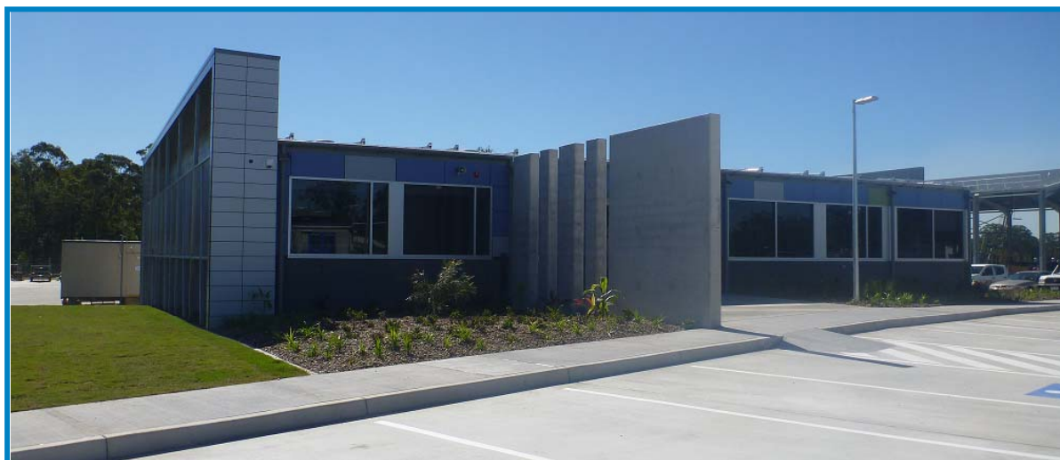
Image 3: Expanded, upgraded office & facilities at the Landsborough CPS project, completed July 2012.
