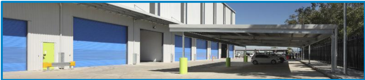
Image 4: Workshop areas and undercover working area underway at the Geebung site redevelopment.
