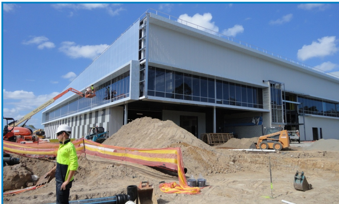
Image 10: Construction progressing at the Geebung Redevelopment Project site.
