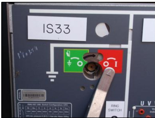
Overtravel resulting in indeterminate position
