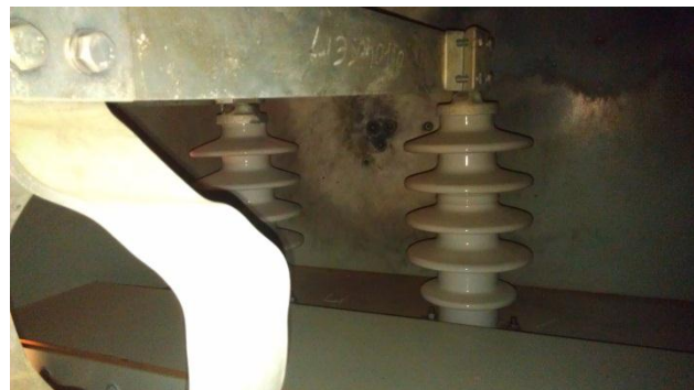
SSIPS Flashover in TRF cable box
