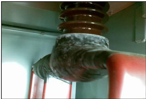
SSGVN Degraded joints
