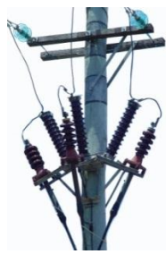
33kV Metal Clad U/G Terminations
