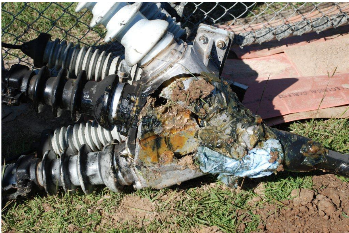
Figure 4 - Explosive Failure - 11kV Pot Head
