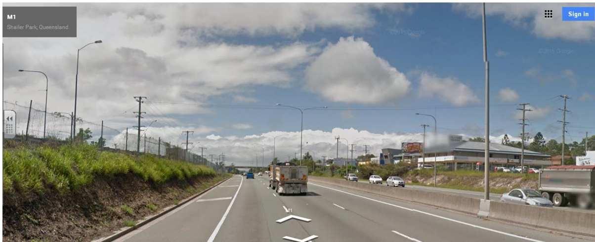
Figure 10: F419 crossing over the Pacific Motorway (M1)
