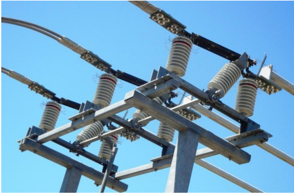
Figure 1: Typical 33kV ABS Isolator in the Switchyard
