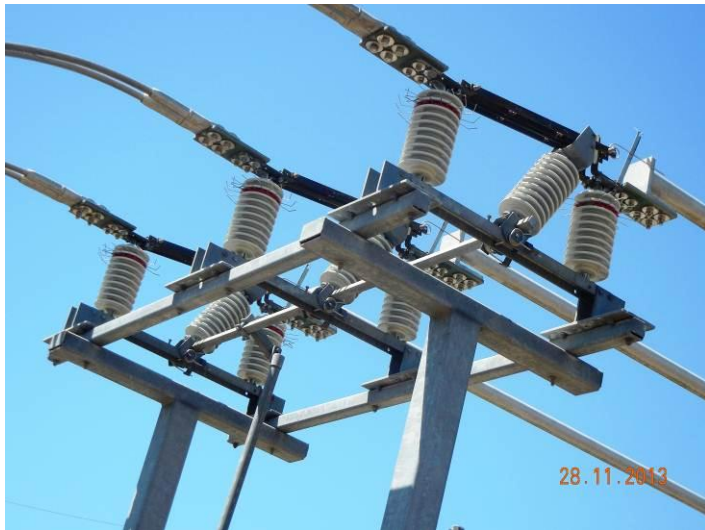
Fig 1- A typical 33 kV [REDACTED] isolator in switchyard Figure 2- Hairline crack on the support insulator.
