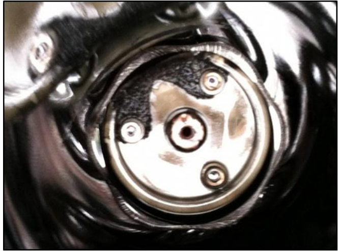
SST114 110kV OCB failure exterior
