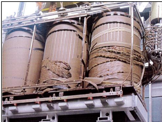
SSCMA winding damage
