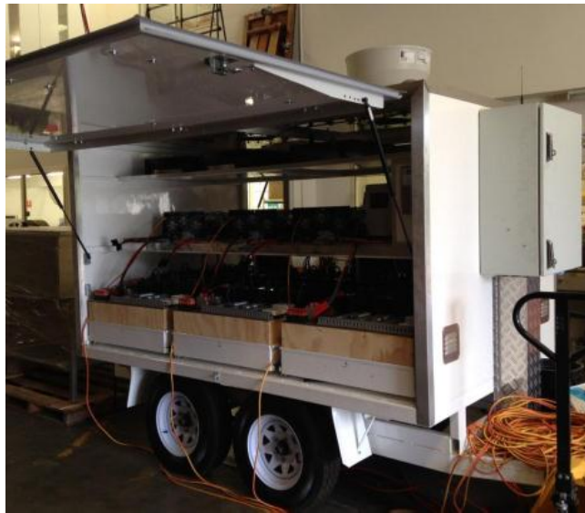
Figure 1: Trial unit - Trailer fitted with batteries, STATCOMs and auxiliary gear
