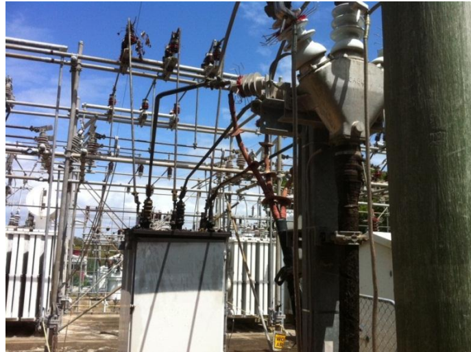
Figure 20: Extent of damage insitu
