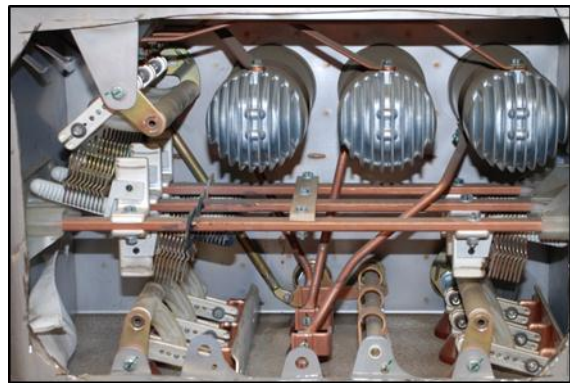
Rear of RMU with overtravel arcing
