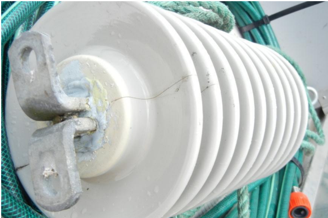
Figure 3: Hairline Crack and the Sealant on the Insulator ABS Insulator from SST16 (Nambour Substation)
