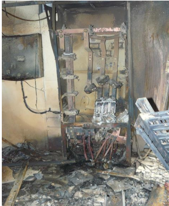
Figure 18: Entry point of LV cables to customer’s switchboard following an incident in the Energex Network
