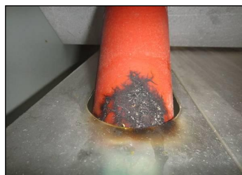
SSCPC Degraded bushings
