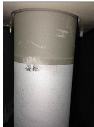
Damaged screen SSLYT CB1T32
