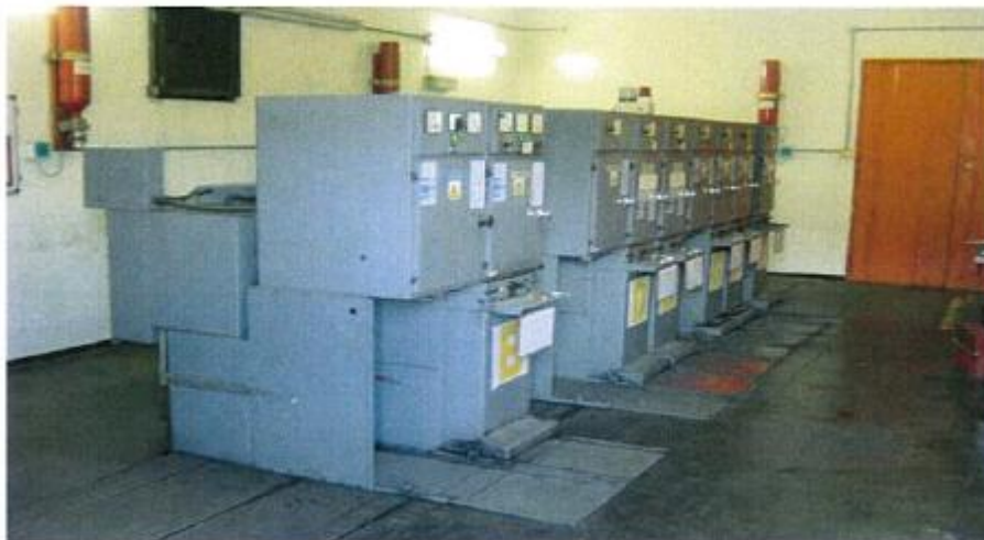
Figure 1: Circuit breakers pre-fault of a manual operation (South Africa)
