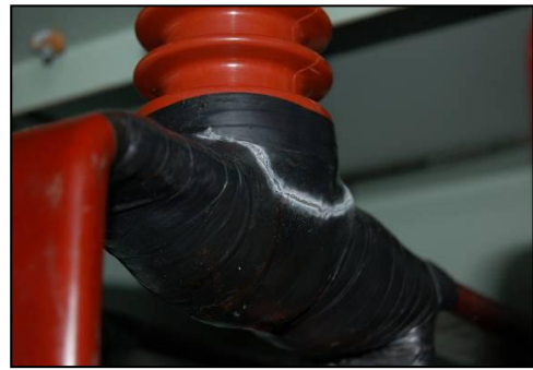
SSRBA degraded joints
