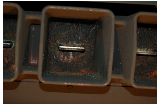
SSMFD Catastrophic CB failure
