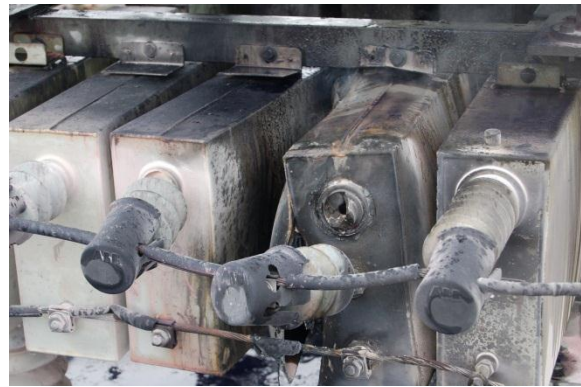
Capacitors from SST108
