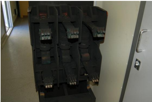
SSMFD Catastrophic CB failure
