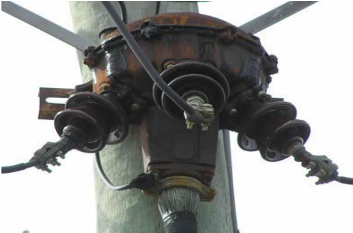
Figure 2 - 11kV Pot Head In Service
