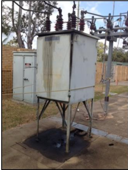
SSLTN 11kV OCB failure exterior
