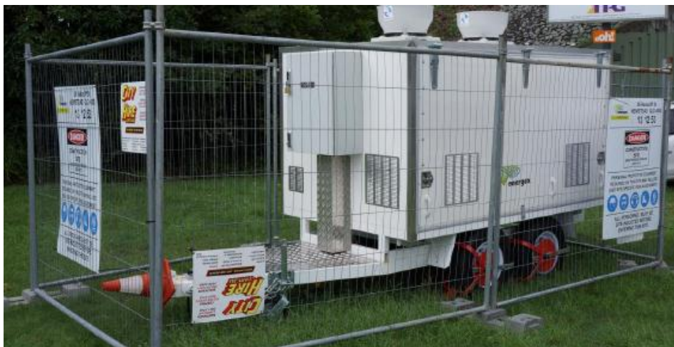
Figure 2: Trial unit - Trailer in service at trial site [REDACTED]
