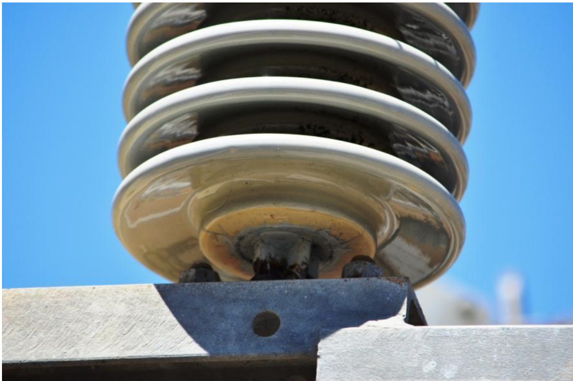
Figure 4: Signs of Pin Corrosion on the Bottom Side of the Isolator Insulator – T136 (Abermain Substation)
