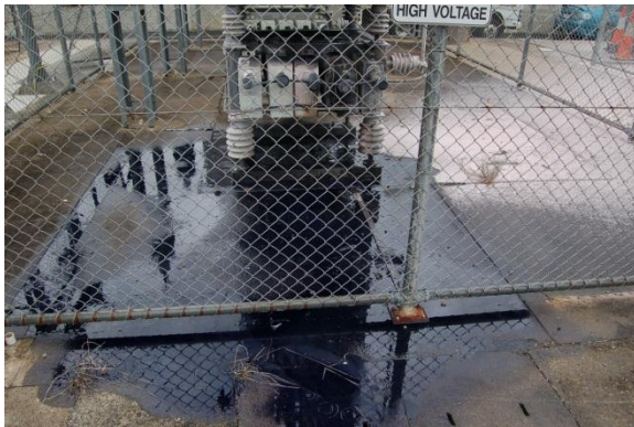
Failure of capacitor bank at SST108
