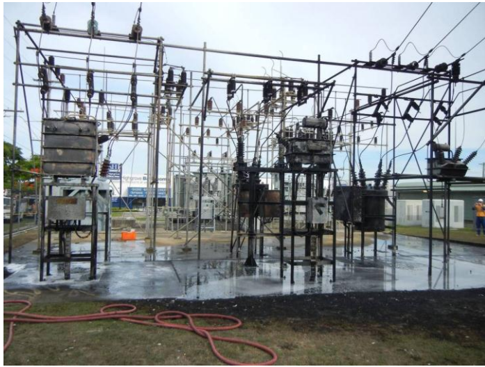
Figure 11: Station Transformer TR8 exploded and expelled 400L of hot insulating oil igniting spontaneous fires
