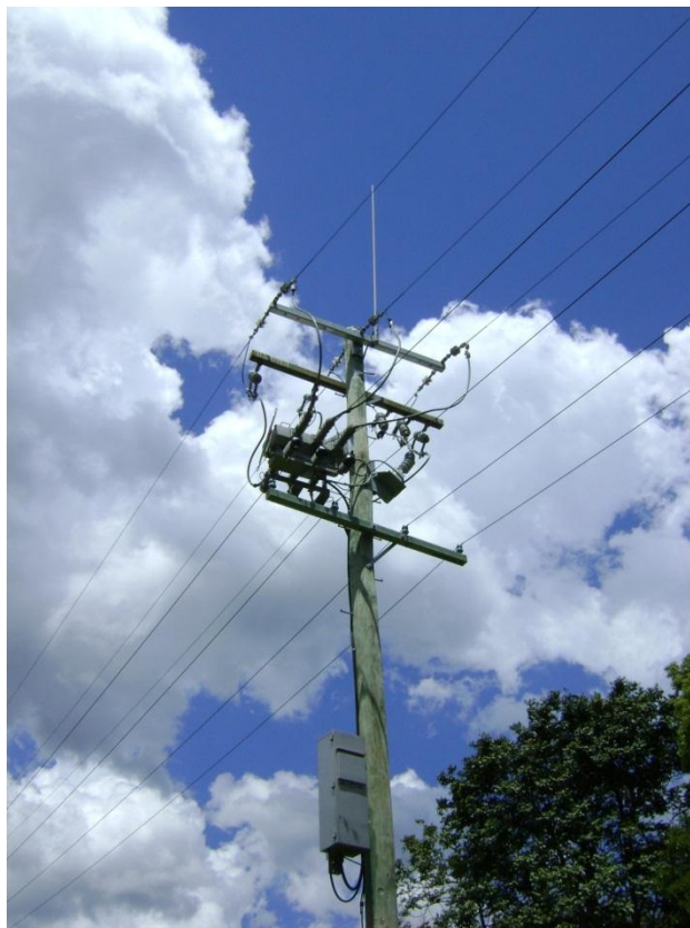
Figure 1: Remotely Controlled Load Break Switch (Side Mount) with Auxiliary Supply VT, Controller and Radio Antenna
