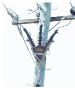
11kV Metal Clad U/G Terminations
