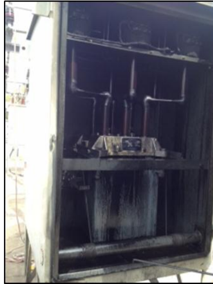
SSLTN 11kV OCB failure internal view
