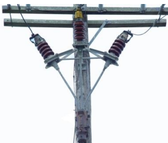
33kV Metal Clad U/G Terminations
