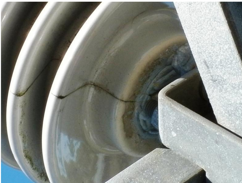
Figure 2: Large Crack on the Underside of an ABS Insulator from SST16
