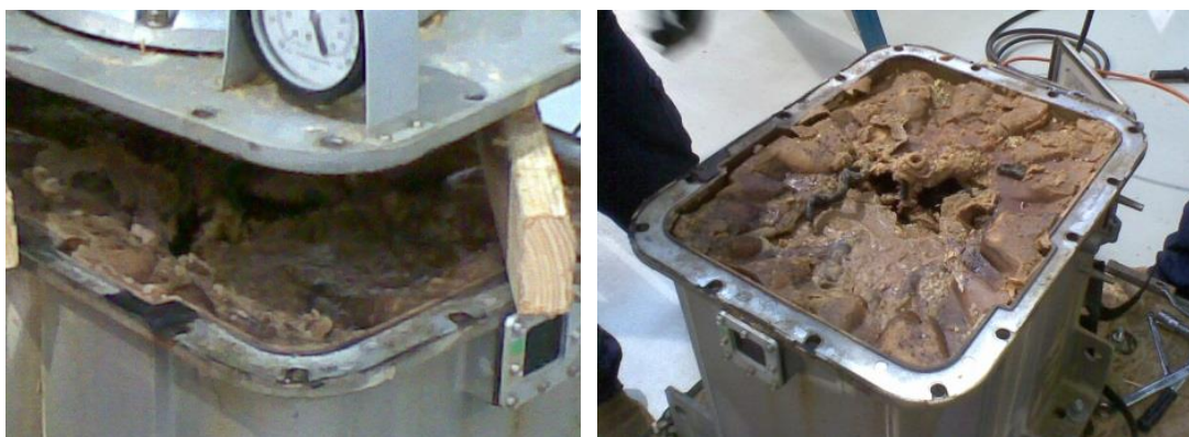
Figure 6: Poor Condition CVT 1
