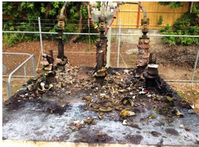
Figure 21: Extent of damage to all 6 bushings of the failed circuit breaker
