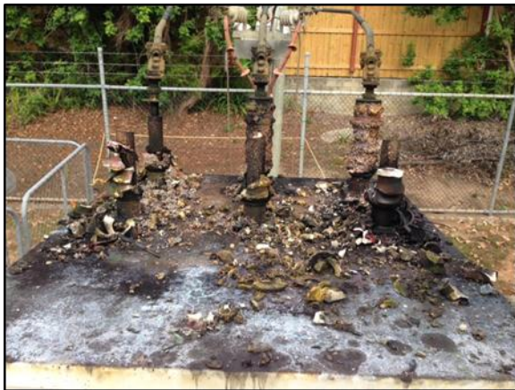
Destruction of bushings at SSLDR
