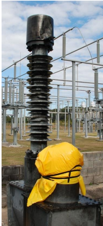
Figure 1: Surrounding Equipment after VT Failure at Mooloolaba
