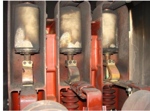
SSCLM [REDACTED] vacuum bottle failure
