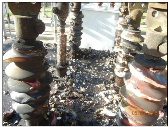
SSLTN Destruction of bushings
