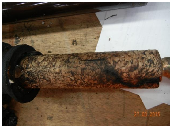
SSLTN tracking due to water ingress
