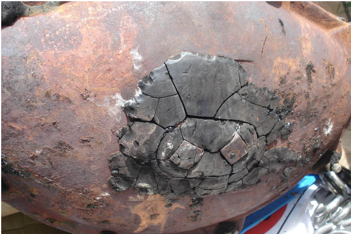
Figure 5 - 11kV Pot Head Leaking Bitumen
