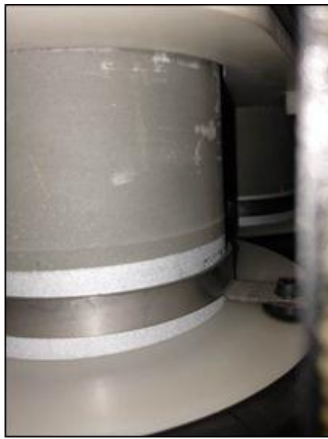
Damaged screen SSLYT CB1022
