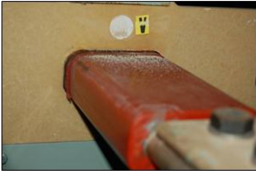
SSCVL Damaged earth screen
