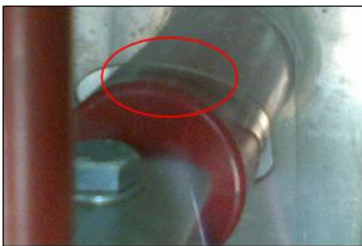
SSBTA Problematic high stress air gap
