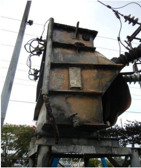
Figure 11: Station Transformer TR8 exploded and expelled 400L of hot insulating oil igniting spontaneous fires
