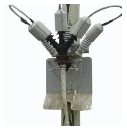
11kV Metal Clad U/G Terminations
