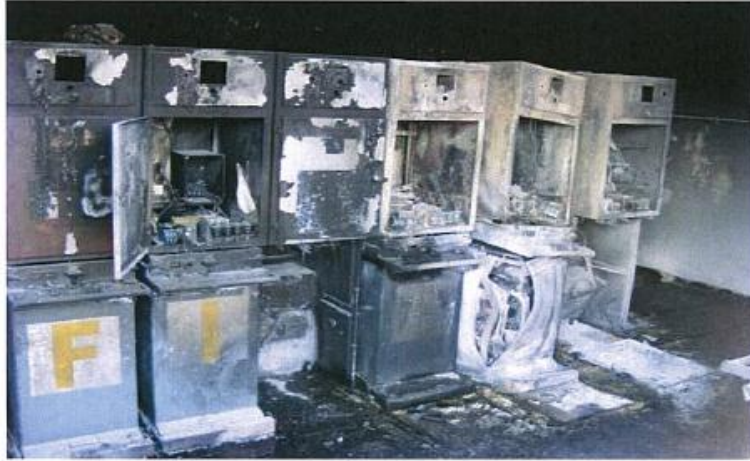
Figure 2: Circuit breakers post-fault of a manual operation (South Africa)
