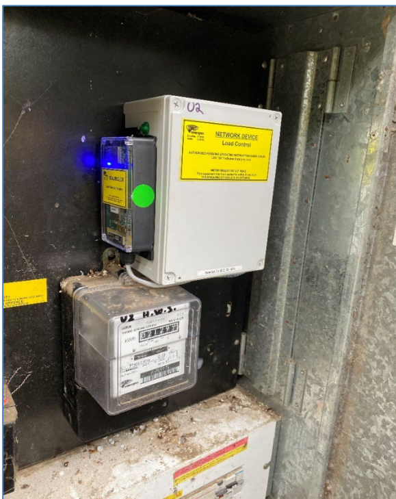
Load control relay and comms device in-situ
