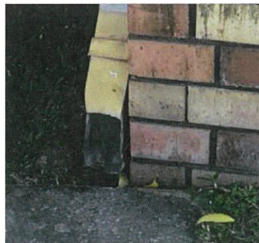
Figure 7: Stormwater downpipe isn't connected to protect footings from movement
