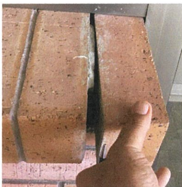
Figure 3: Deteriorated brick wall mortar joints due to age
