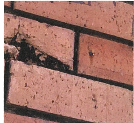
Figure 2: Deteriorated and cracked bricks (external wall)
