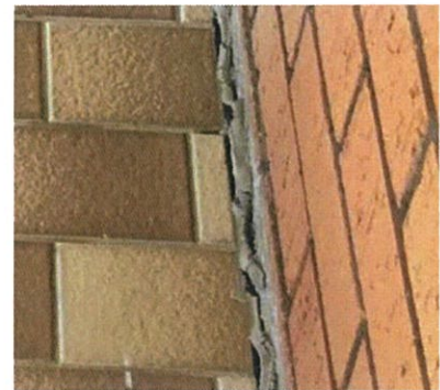
Figure 8: External paths moving away from wall due to excessive moisture
