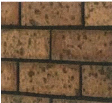
Figure 6: Water absorbing classroom brickwork
