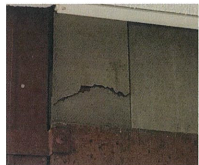
Figure 5: Edge concrete bond beam has expansion cracking from reinforcement corrosion, reducing tie down capability. Structurally inadequate for cyclone area.
