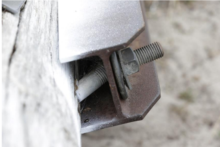
Figure 8: Example of a bolted reinforcement connection in bending.
