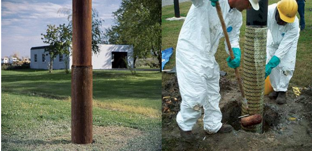
Figure 4: Example of a finished and during-application wrapped type reinforcement.
