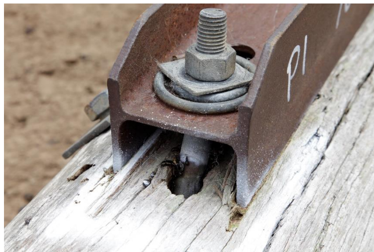
Figure 9: Example of the timber being deformed by a bolted connection.
