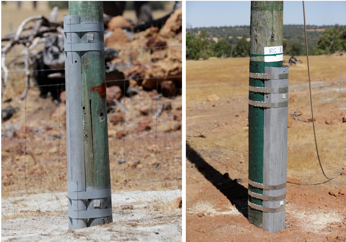
Figure 1: Examples of Banded reinforcement.
