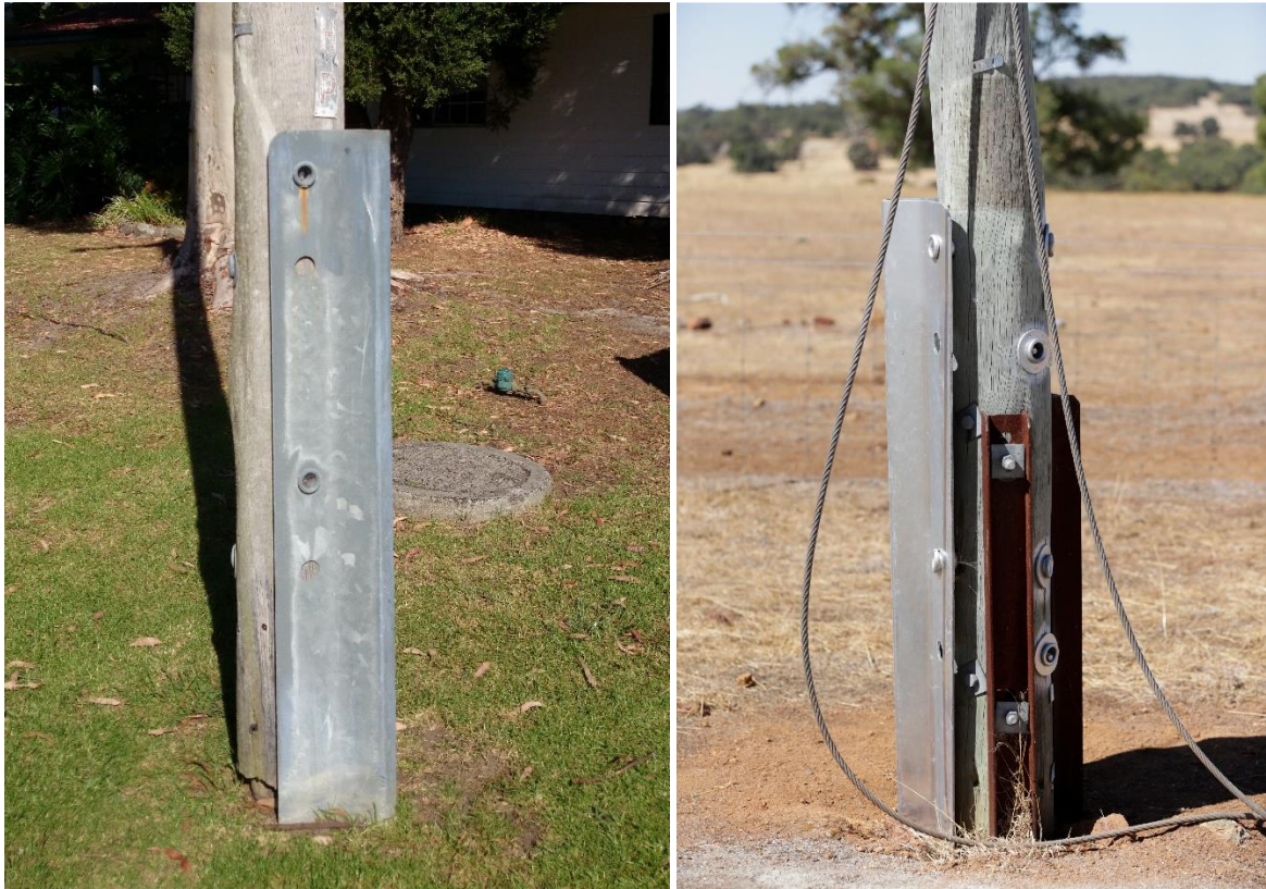
Figure 2: Examples of Bolted reinforcement types.
