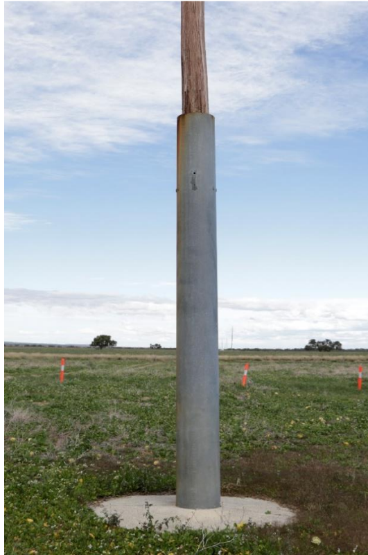
Figure 3: Example of a Rebutted pole.
