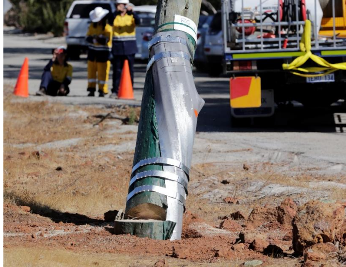
Figure 6: An example of the severe deformations that are normally required before bands are overloaded, if they are installed correctly. Typical of banded reinforcement loaded in the strong direction.
