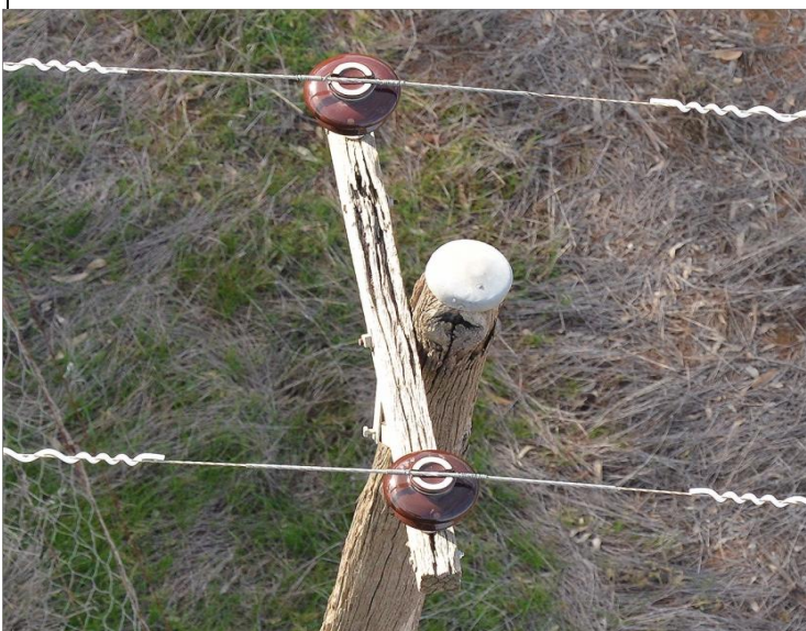
Crossarm deteriorated, deep cracks, weathered – A3 task
