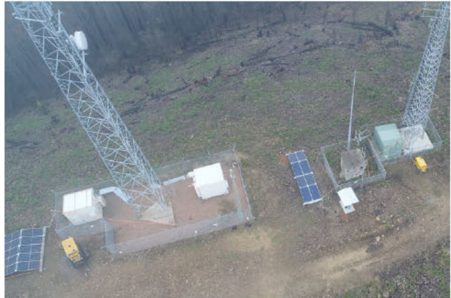
Figure 4 Peak Alone temporary SAPS installations – March 2020
