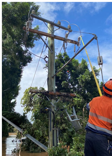
Figure 6: Safety works near Lismore
