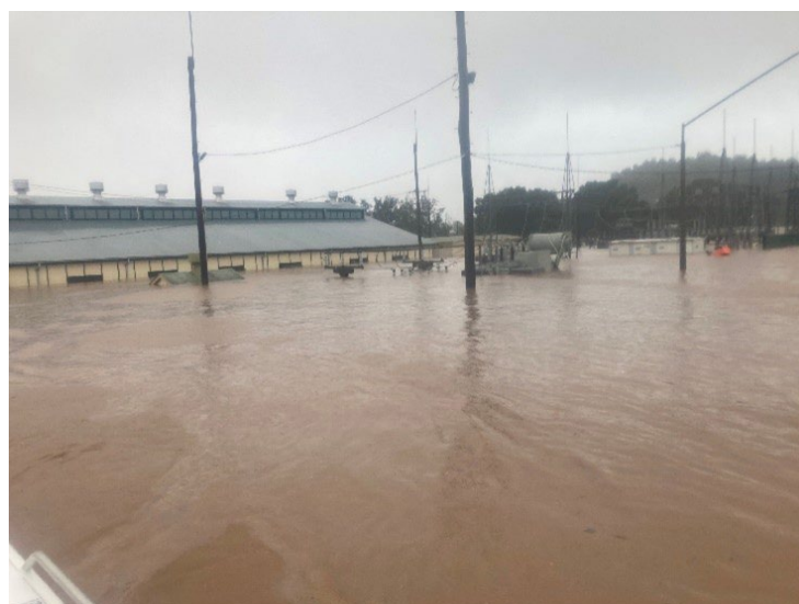
Figure 8: Zone substation and depot inundation
