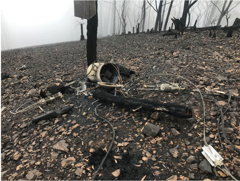
Photo – The remnants of the transformer and pole that fed Peak Alone Communications towers.
