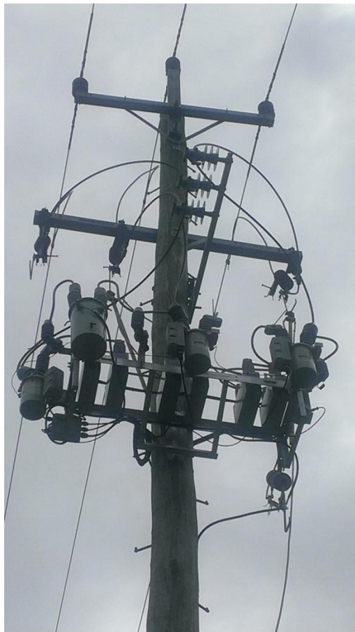
Figure 3 - Clarendtown trial capacitor bank installation
