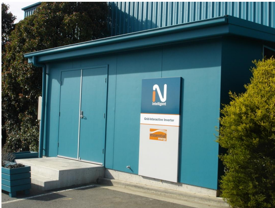
Figure 1 Queanbeyan Inverter Installation
