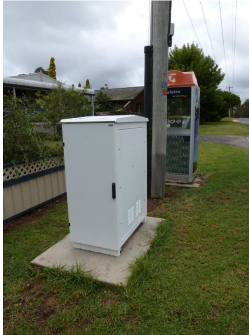
Figure 2 Bega / Kalaru Inverter Installation
