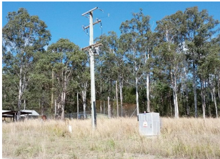
Figure 3 Pappinbarra Inverter Installation
