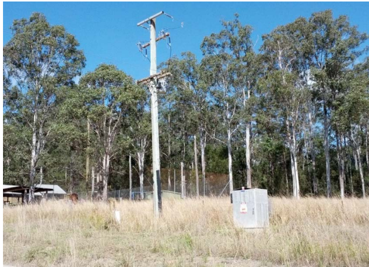
Figure 5 Pappinbarra Inverter Installation
