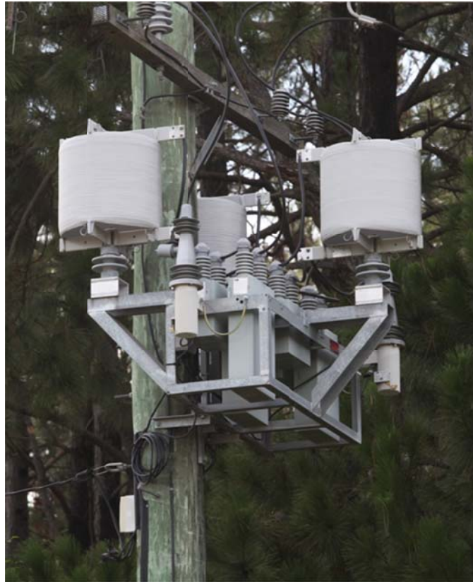
Figure 13 - Pole Top Capacitor
