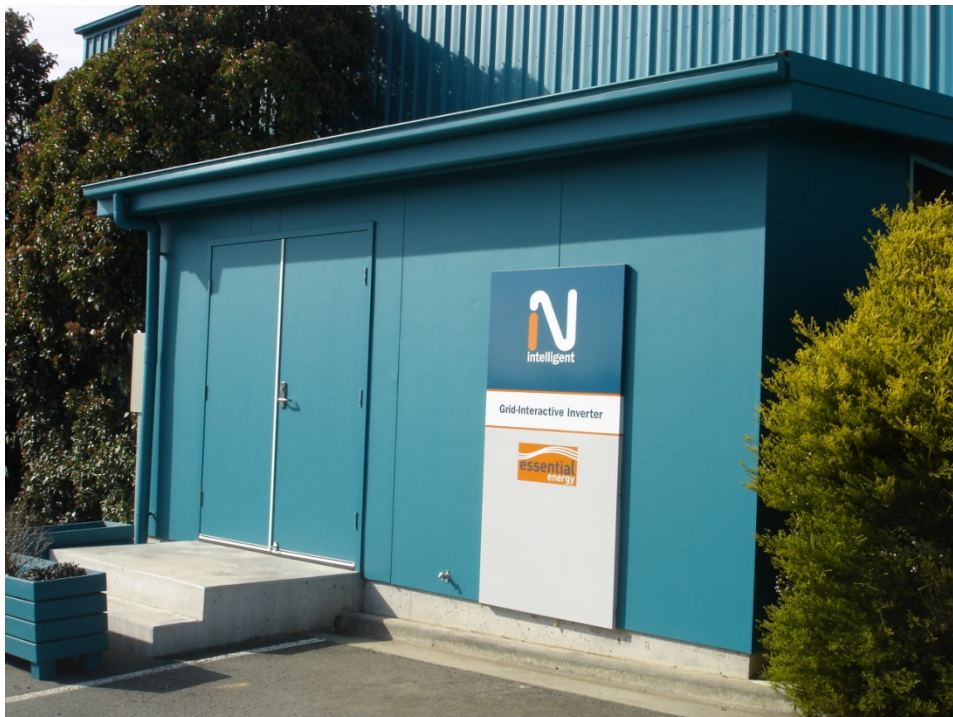
Figure 1 Queanbeyan Inverter Installation
