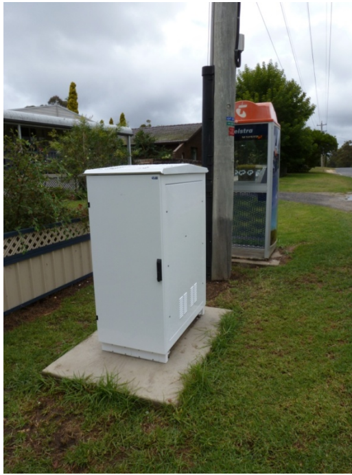
Figure 3 Bega / Kalaru Inverter Installation
