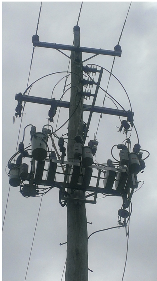
Figure 15 - Clarencetown trial capacitor bank installation
