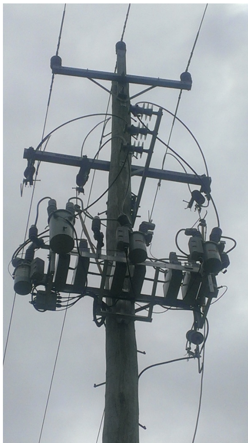
Figure 14 - Clarencetown trial capacitor bank installation
