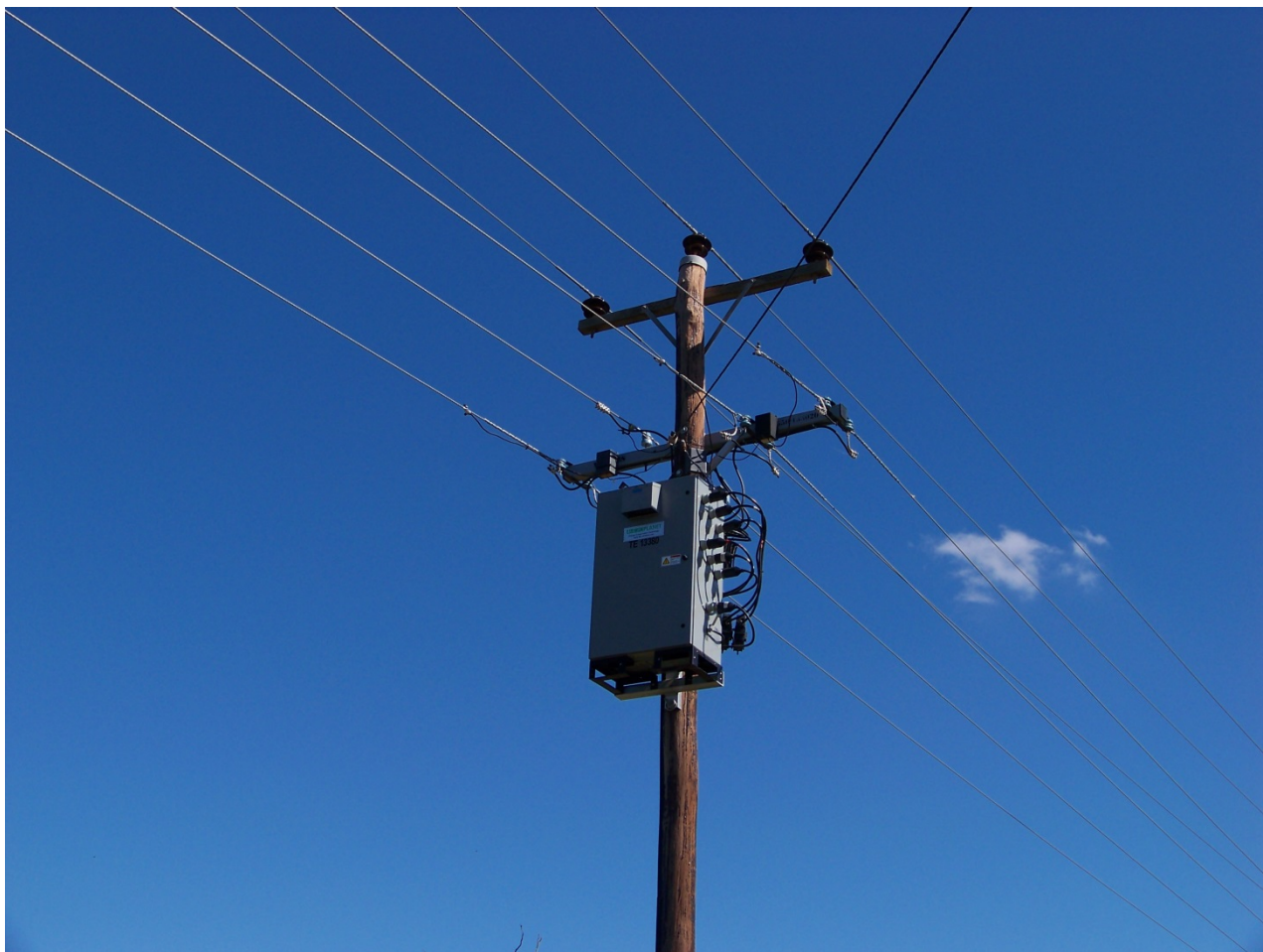
Figure 10 - Low Voltage Regulator
