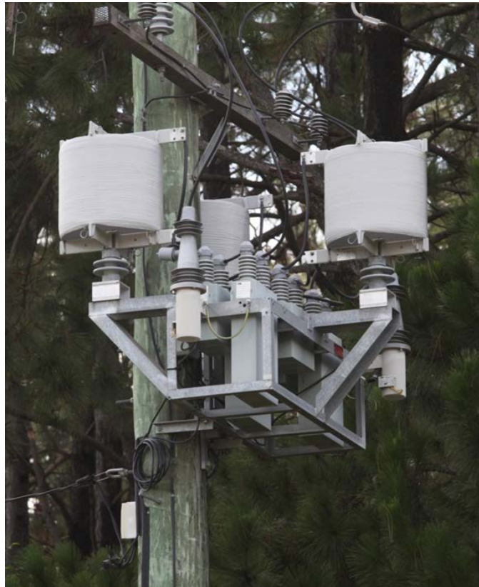
Figure 12 - Pole Top Capacitor
