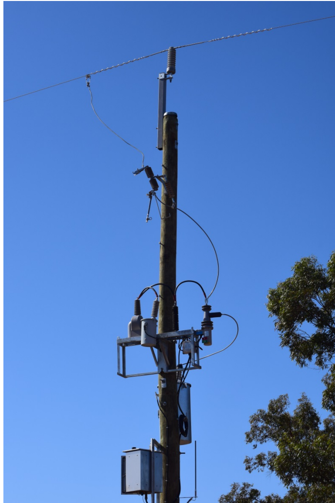
Figure 17: Nyngan SWER Switched Reactor
