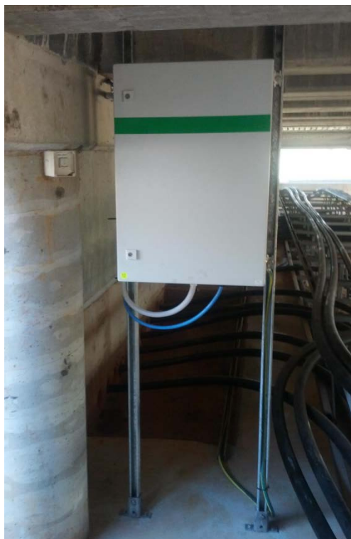
Figure 8 - Clearwater Zone Substation 5kVA four quadrant inverter (atypical) installation
