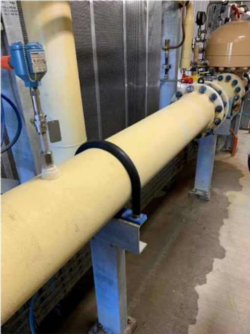
Very limited space to install the meter inside the PRS enclosure. If install in the enclosure, accuracy of the meter be affected and the accuracy won't be known until the meter is installed. It also affect the operation of the PRS regulator
