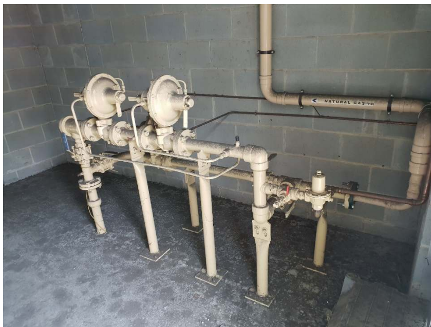
Figure 2: Secondary Boundary Regulator in the New Section to be Upgraded
