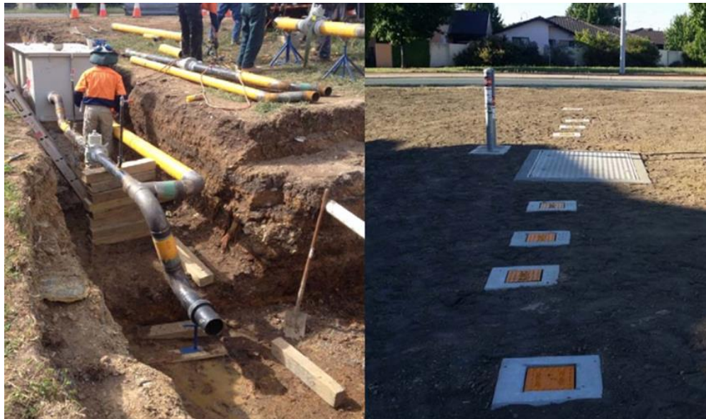
Figure 3.9 Installing a new secondary district regulator set (before and after).
