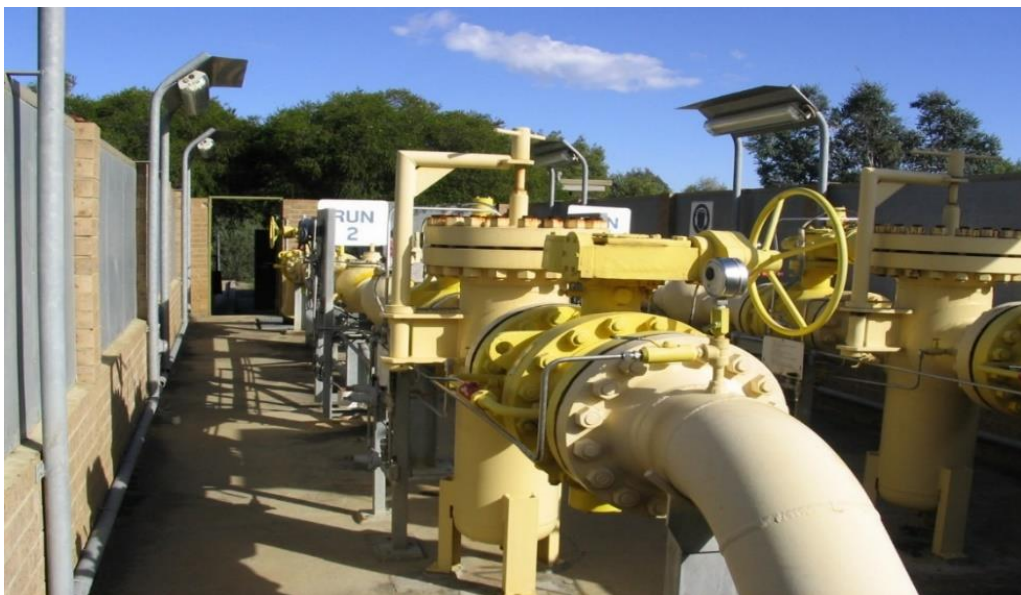
Figure 3.7 Inside the current Watson high pressure gas facility
