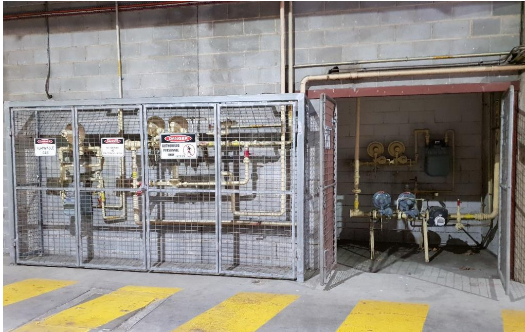
Figure 3.8 Shopping centre regulators and piping to be upgraded
