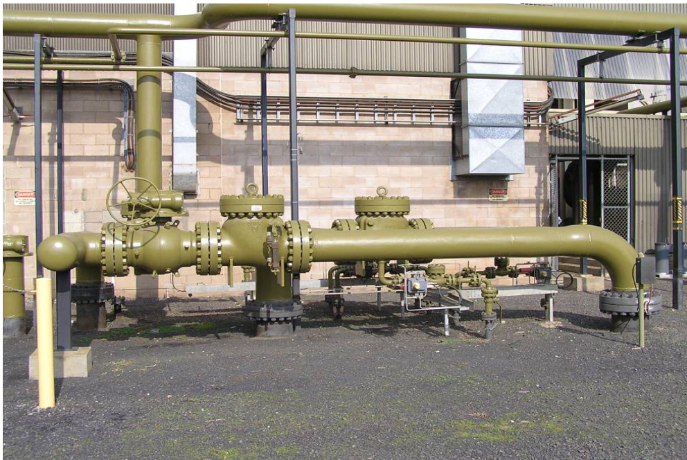
Photo 21: Brooklyn station pipework adjacent to stage two building
