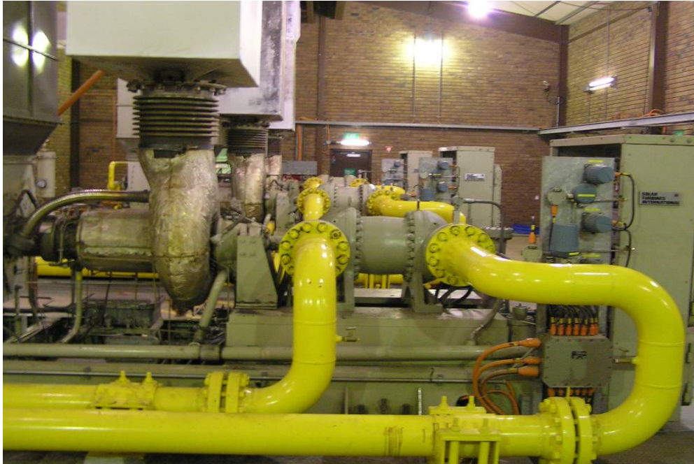
Photo 26: Wollert Saturn compressors
