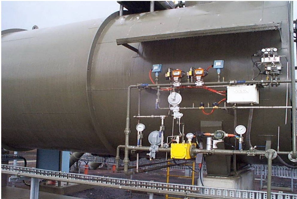
Photo 16: Brooklyn high-pressure water bath heater adjacent to stage three building
