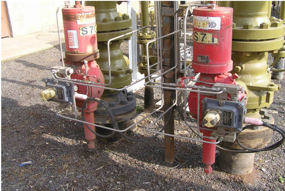
Photo 20: Brooklyn Saturn unit isolation valves
