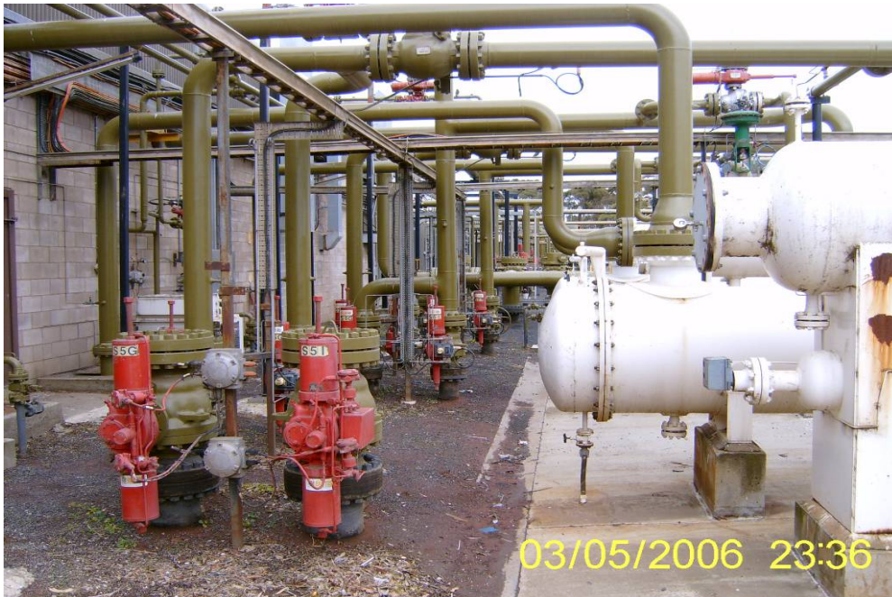
Photo 4: Saturn unit isolation valves, inlet scrubber and watercooled exchanger
