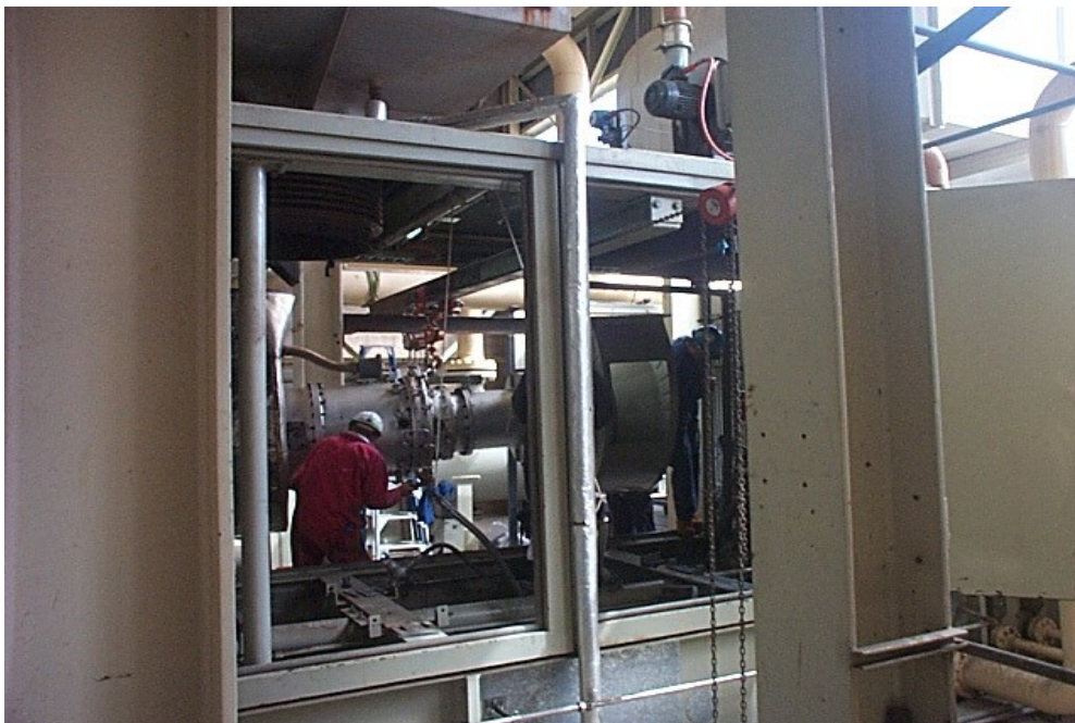
Photo 11: Brooklyn Centaur package in stage three building showing interference with building support piers and congestion with processing equipment adjacent to hot services.
