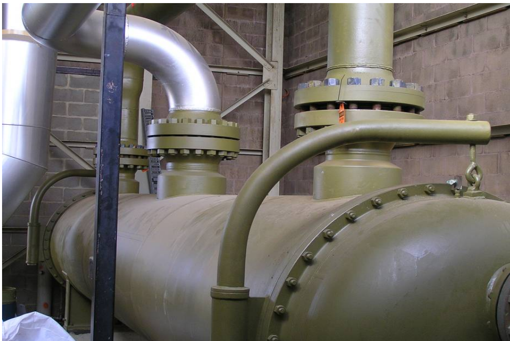
Photo 19: Brooklyn stage three building showing high-pressure watercooled exchanger adjacent to Centaur unit 11
