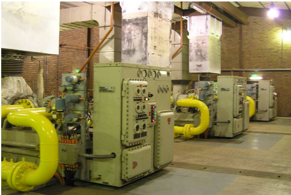
Photo 25: Wollert Saturn T1200 compressors in compressor building
