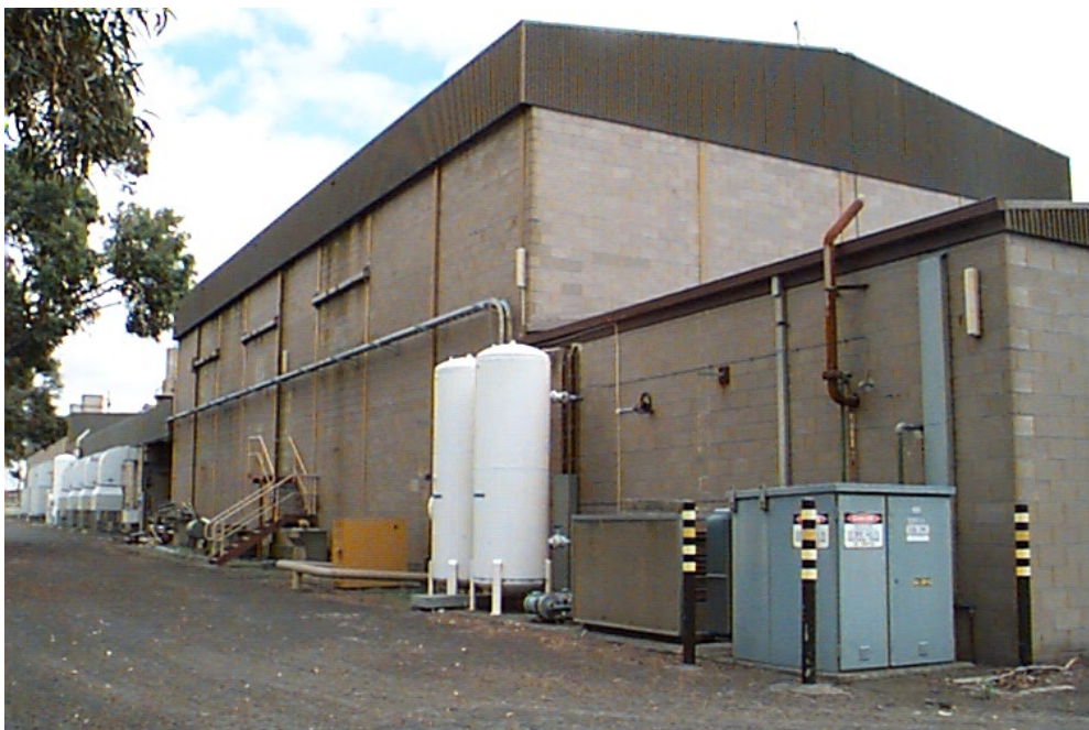
Photo 7: Rear of stage one building, with air receivers in foreground
