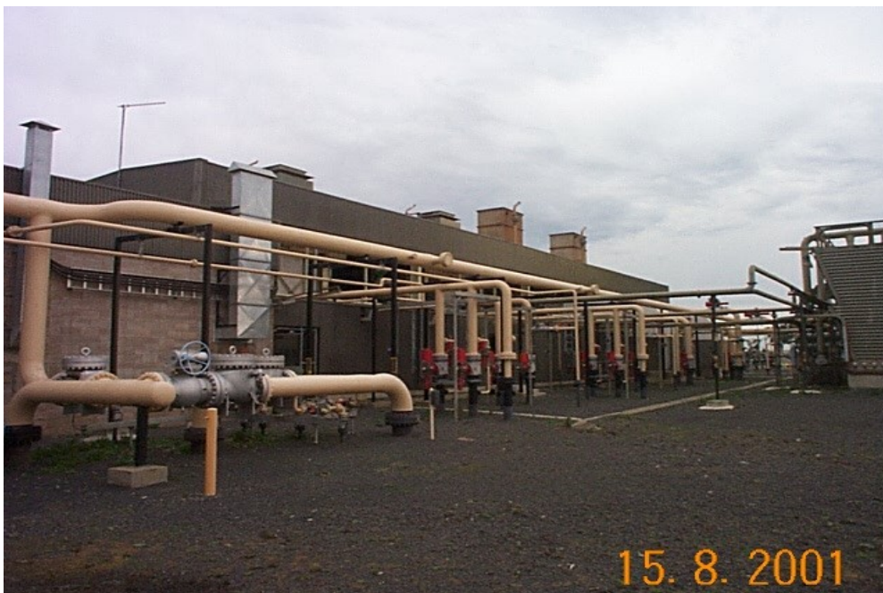
Photo 9: Brooklyn, stage two building with congested pipework and cooling towers in foreground
