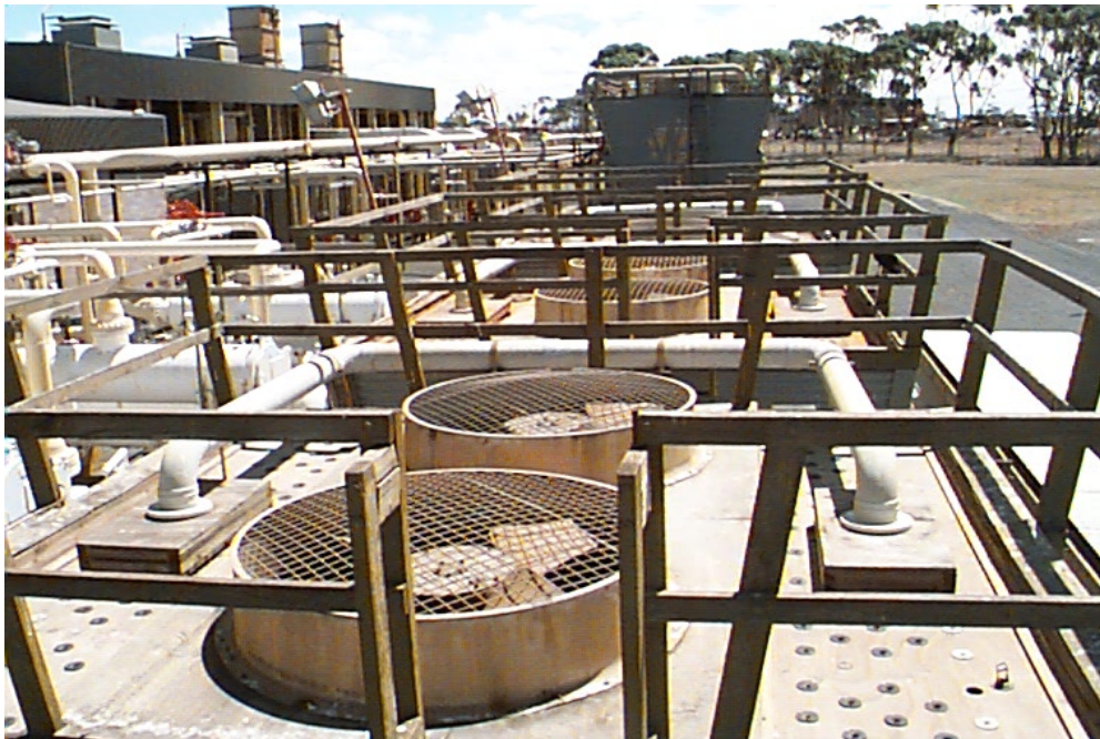
Photo 2: Brooklyn cooling towers
