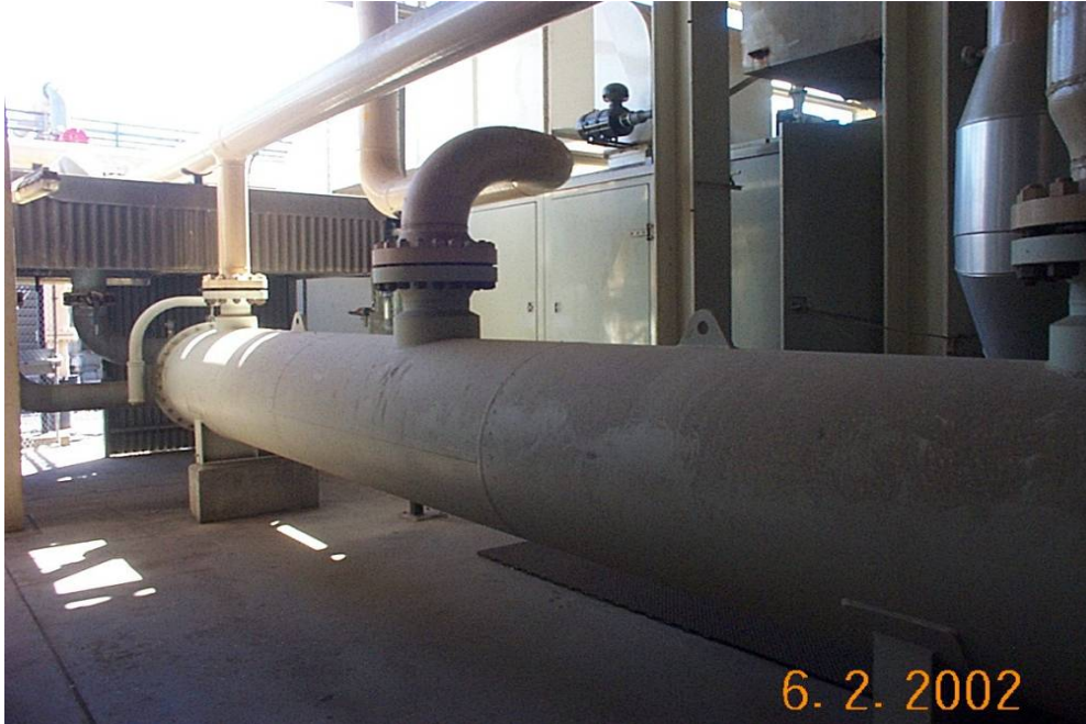
Photo 10: Brooklyn Centaur 11 and watercooled exchanger in foreground, showing congestion of process equipment which interferes with maintenance
