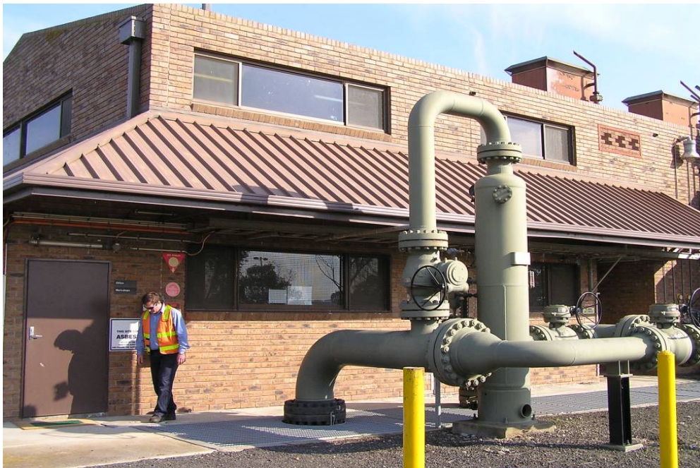
Photo 23: Wollert station inlet suction scrubber
