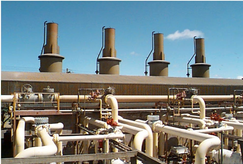
Photo 8: Brooklyn stage 2 building with congested pipework in foreground
