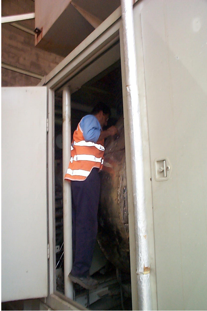
Photo 14: Brooklyn stage 3 standard Solar enclosure
