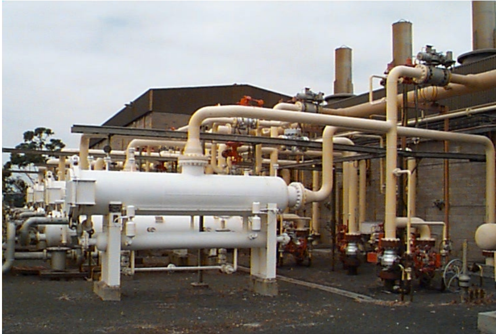
Photo 3: Brooklyn inlet separators and watercooled gas exchangers for Saturns 6, 7, 8 and 9
