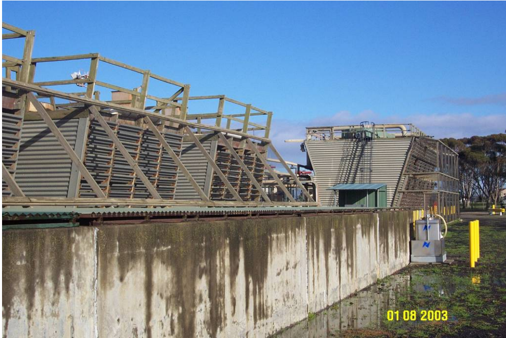
Photo 1: Brooklyn cooling towers
