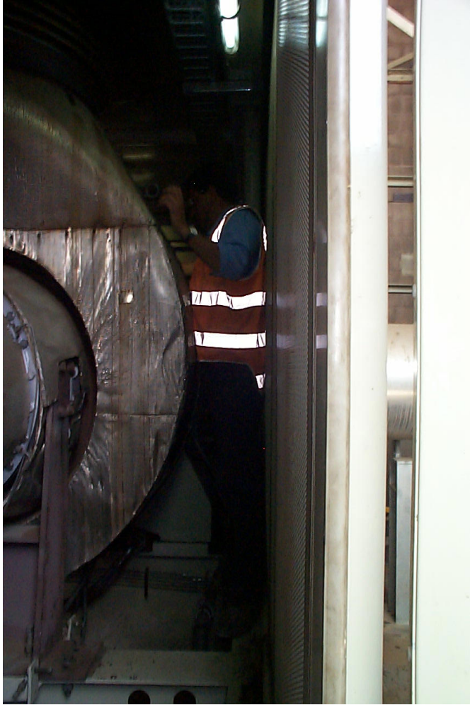
Photo 15: Solar Centaur enclosure
