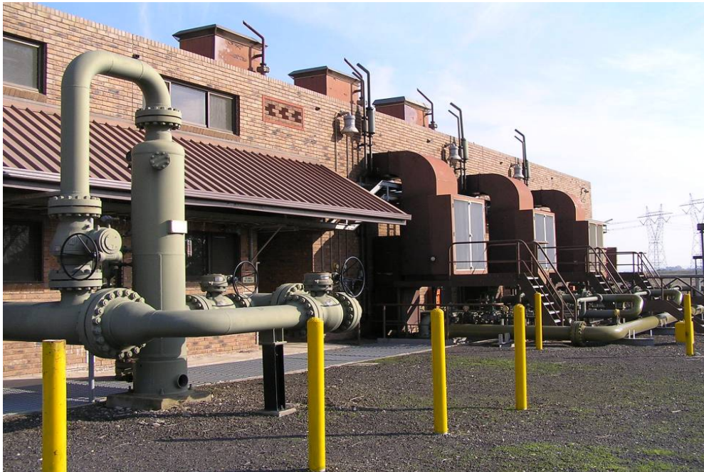
Photo 24: Wollert station and unit piping
