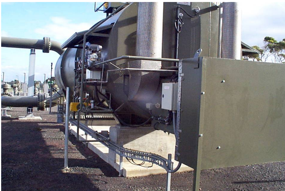
Flue stacks can be seen in the foreground and process gas connections in the background.
