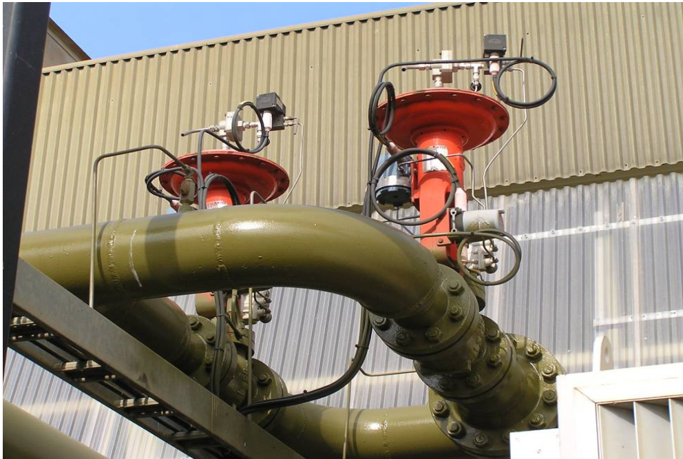
Photo 22: Brooklyn Centaur Unit 11 anti-search valves, adjacent to air inlet
