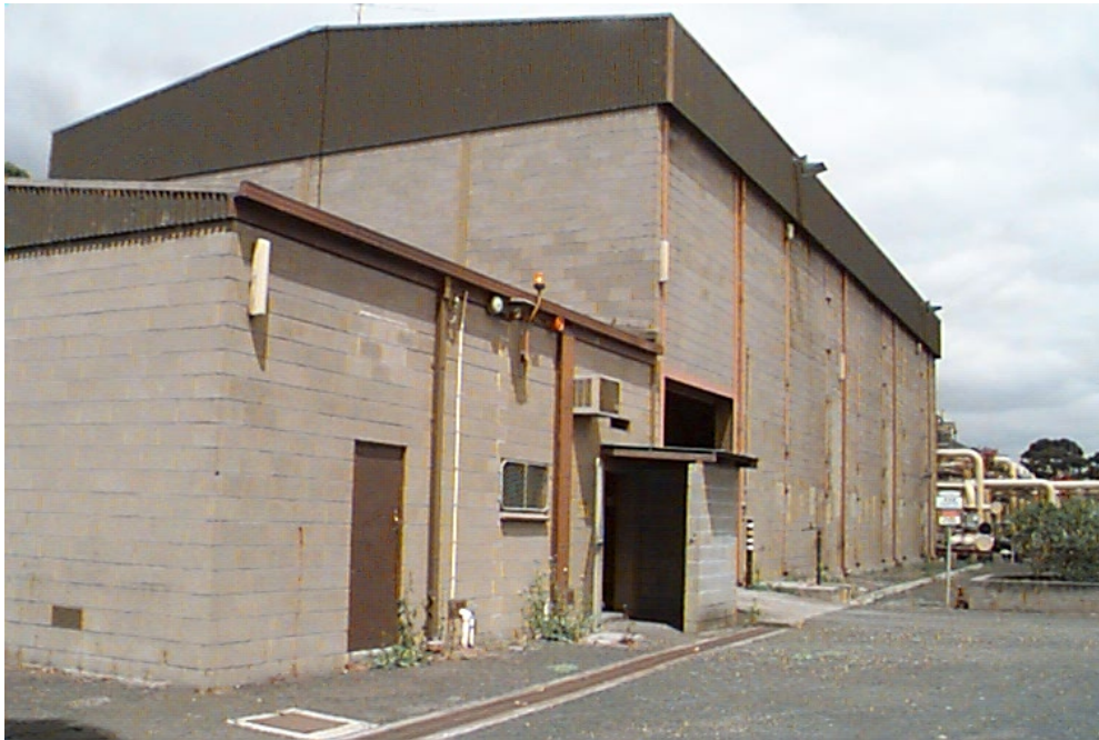
Photo 6: Brooklyn, stage one building, control room in foreground
