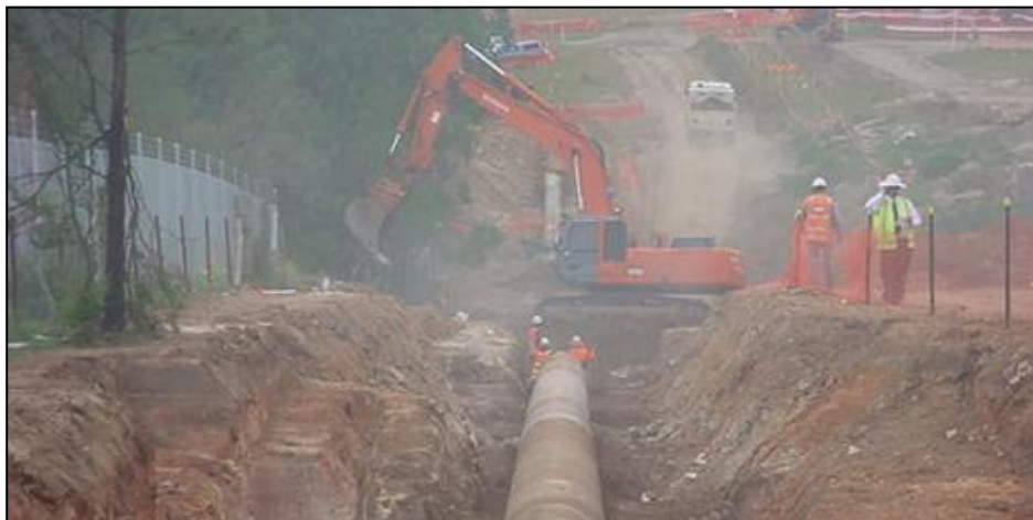
Figure 28 Exposing the Licence 1 pipeline at Simpsons Creek during mine subsidence works
