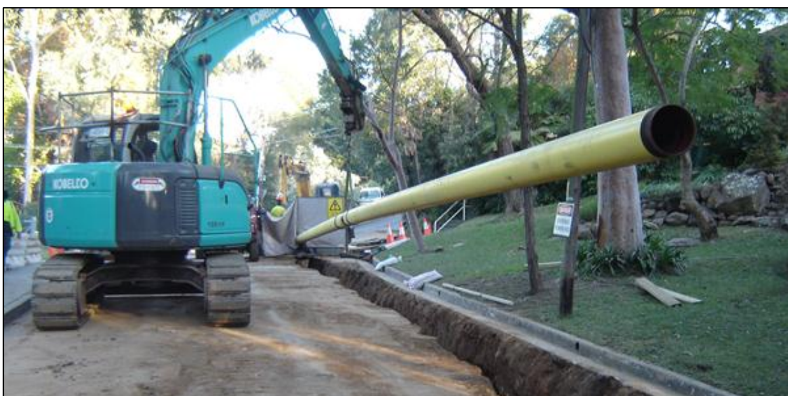
Figure 30 Steel main being laid
