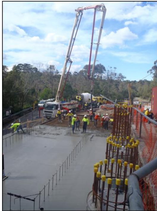
Figure 37 Civil works for construction of Lane Cove PRS
