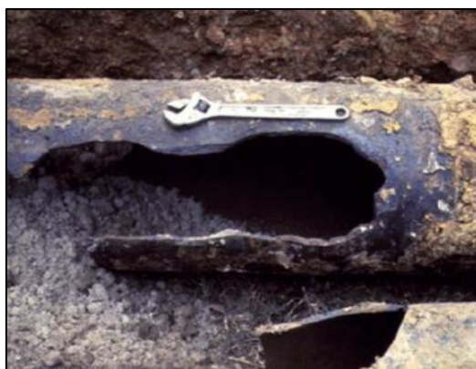
Figure 31 Typical cast iron mains condition prior to rehabilitation
