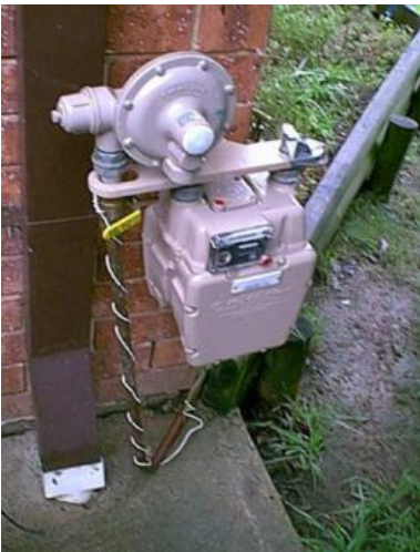
Figure 42 Residential gas meter
