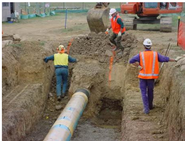
Figure 29 Site preparation for protective works prior to a road crossing
