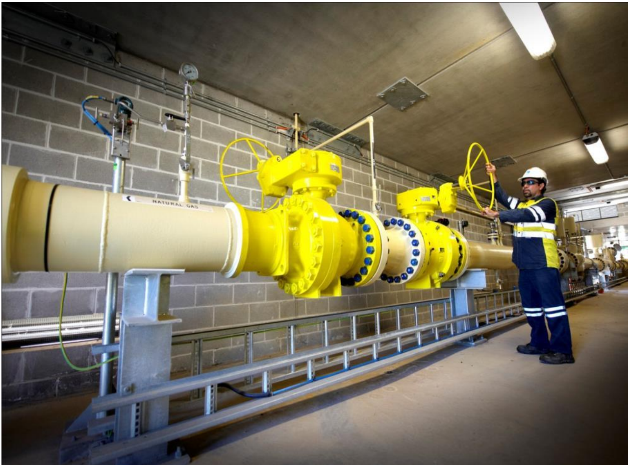
West Hoxton Primary Regulator Station
