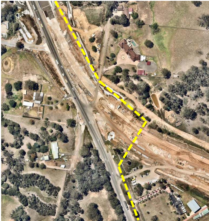
HDD across the new The Northern Rd upgrade
