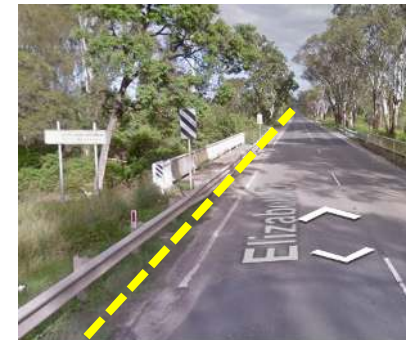
Ground view of Elizabeth Drive with Badgerys Creek crossing requiring either HDD or bridge crossing
