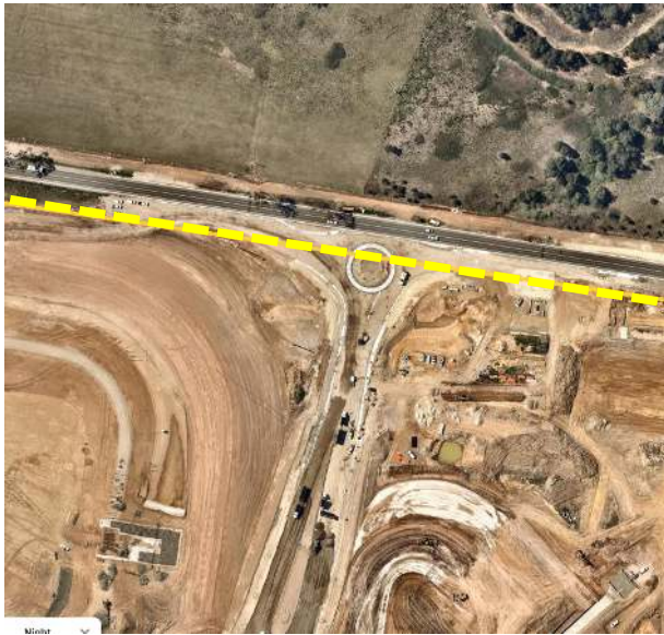
Elizabeth Drive and the second road crossing at the new airport road
