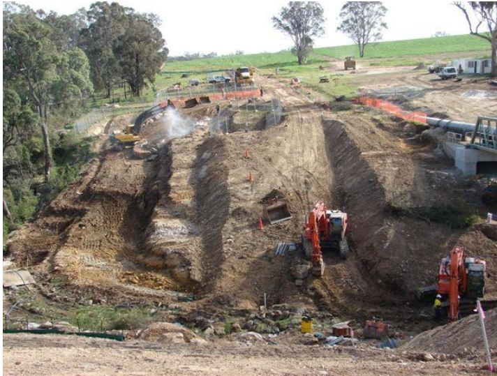
Figure 3 – Excavating the JGN Pipeline at {c-i-c}
