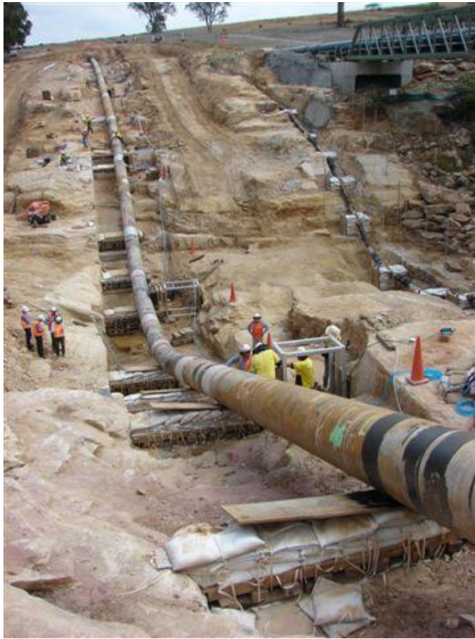
Figure 4 – Stage 2 Mitigation Works on JGN Pipeline at {c-i-c}
