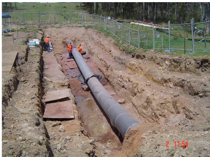
Figure 2 – Stage 5 Rehabilitation of JGN pipeline at Unnamed Creek
