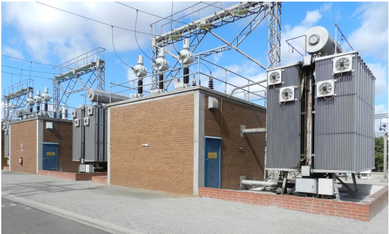
Figure 2–3: BD Transformer Enclosures and Radiators
