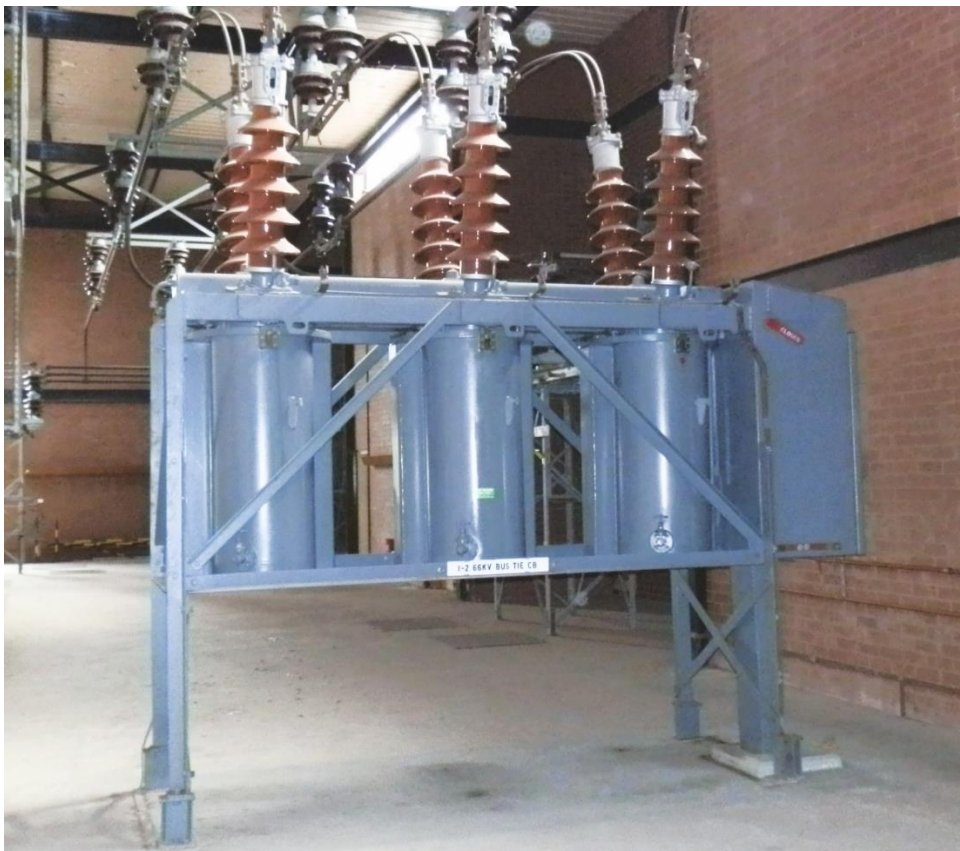
Figure 2–3: CS 66kV Bus Tie CBs
