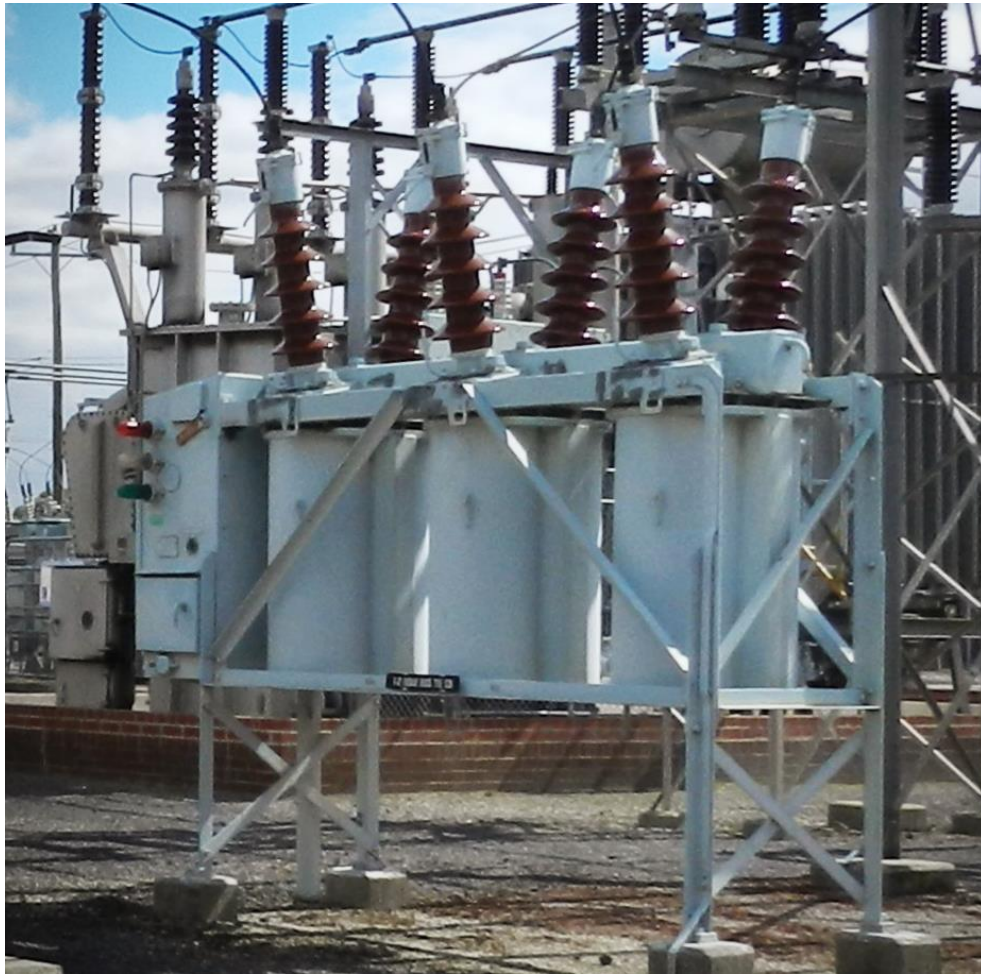
Figure 2–4: CN 1-2 66kV Bus Tie CB
