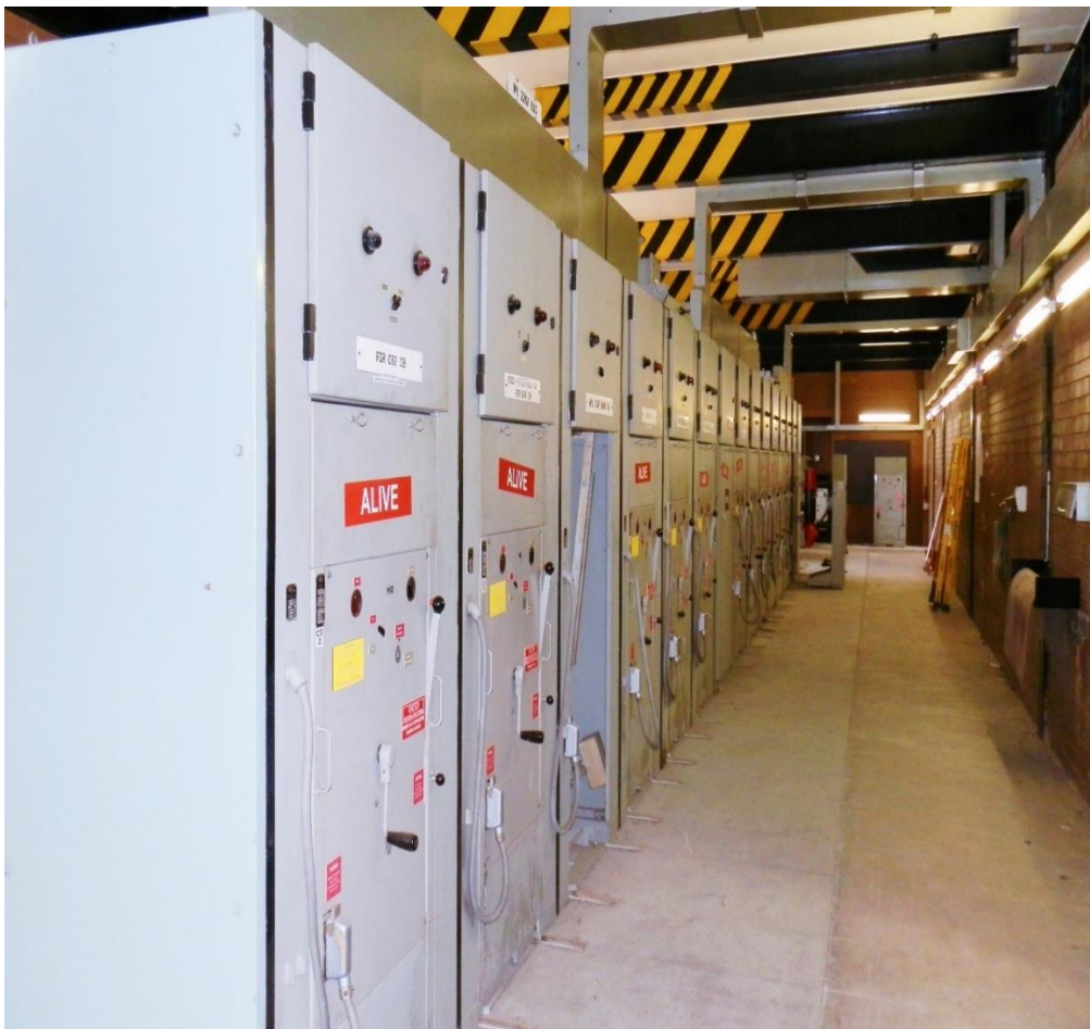
Figure 2–2: CS 22kV Switchgear
