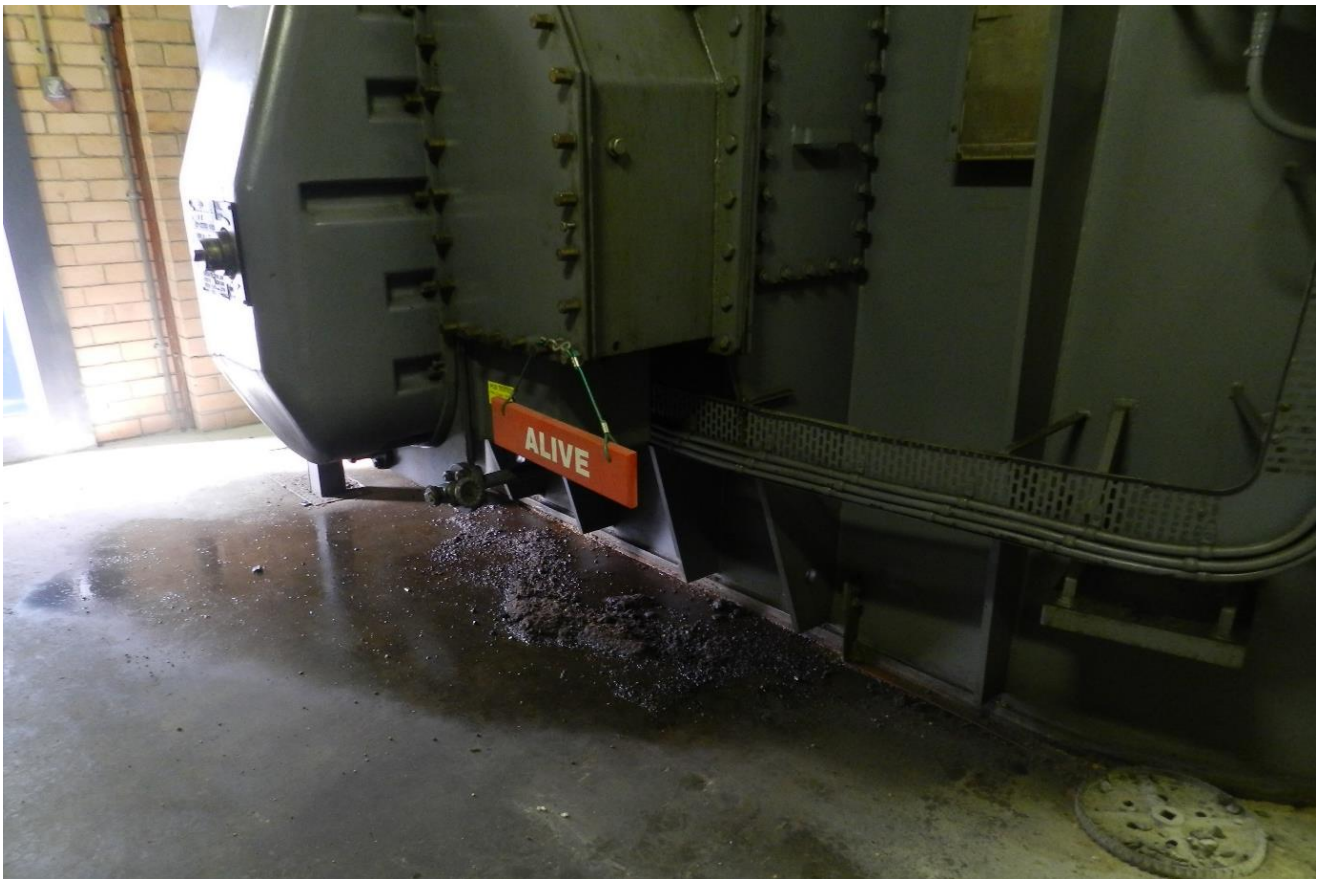
Figure 2–4: No.2 Power Transformer Oil Leaks
