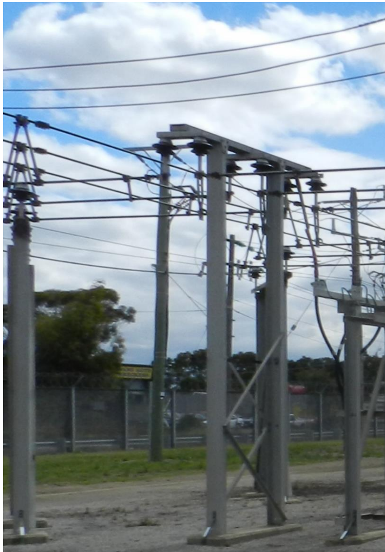
Figure 2–3: CN 22 kV Transfer Bus
